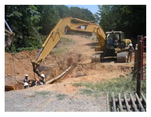
Figure 20 – Worker connecting pipeline sections. Pipeline corridor can be seen in the background.
