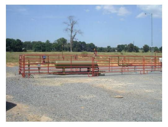
Figure 19 – Gas metering station at a producing well site.
