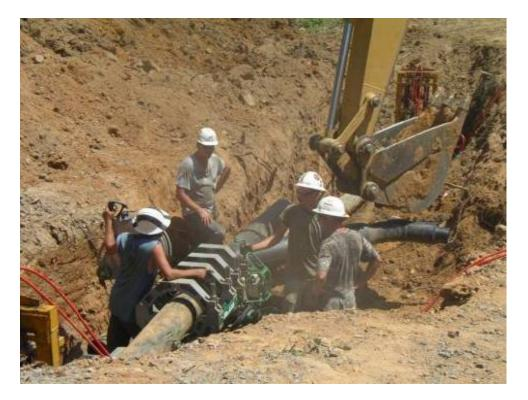
Figure 21 – Workers splicing plastic pipeline and connecting a junction line in the field.
