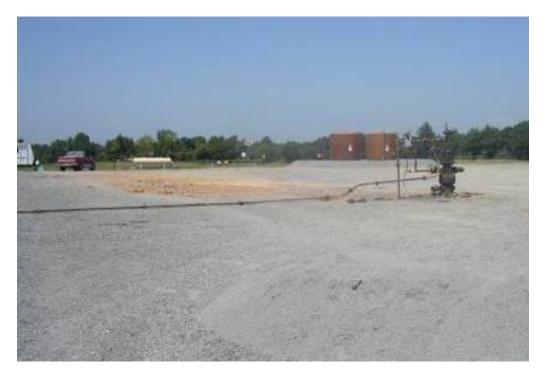
Figure 2 – Newly constructed well showing gravel pad.
