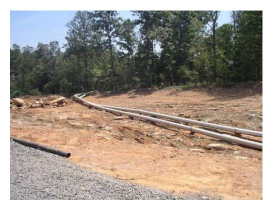
Figure 10 – Water pipeline conveying water for a frac job.
