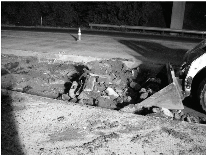
Removal of debris after demolition of a deteriorated pavement slab.
