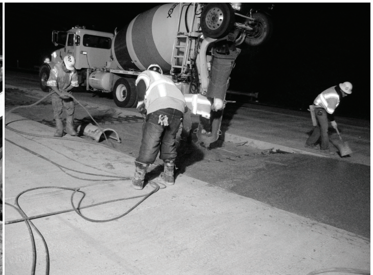
Placement and consolidation of rapid strength concrete in prepared roadbed.
