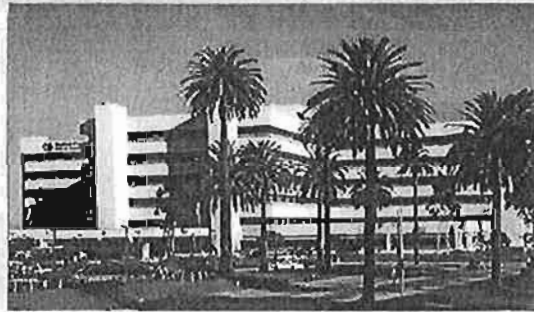
Building 500 (James W. Wadsworth Building) at West L.A. Campus
