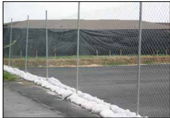
7. Northwest corner of MP. Part of EBES's roof can be seen. The lined fence helps prevent renegade dust and the berm prevents site runoff during cleanup and restoration activities.
