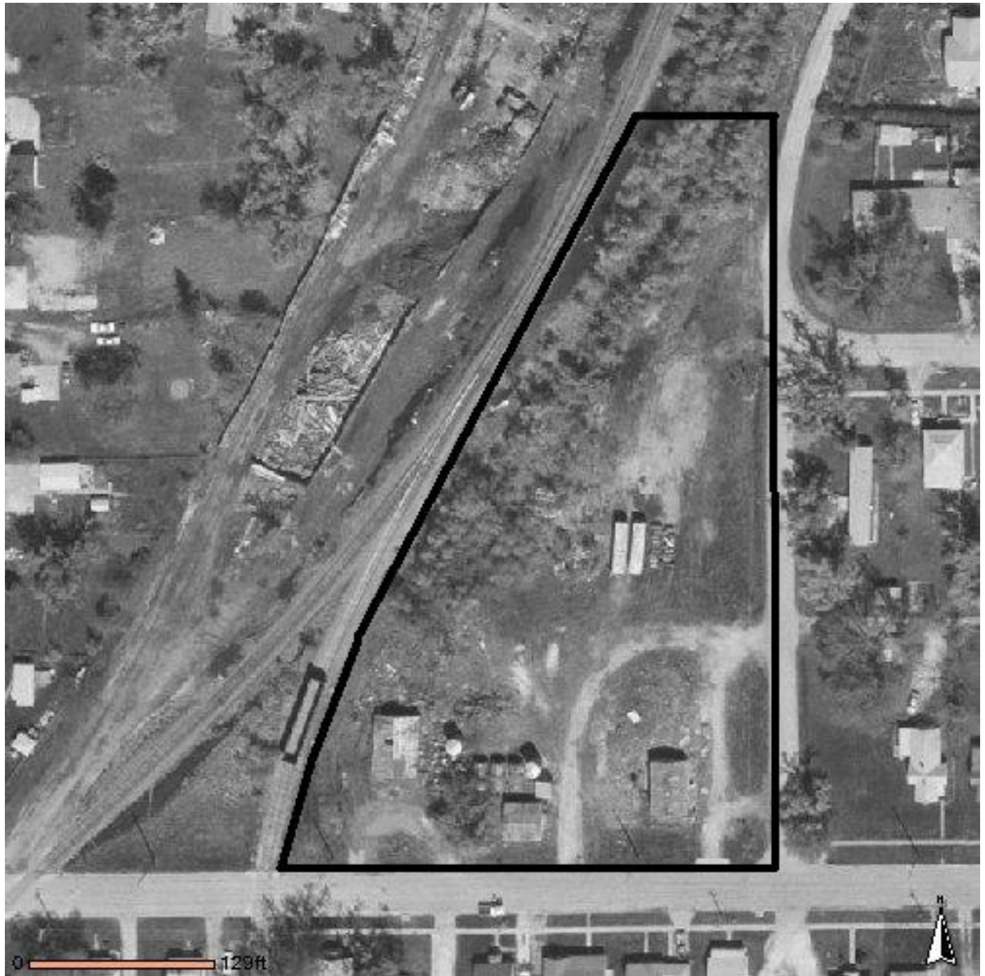
Figure 1 – Aerial View of Site Prior to Removal of Structures
