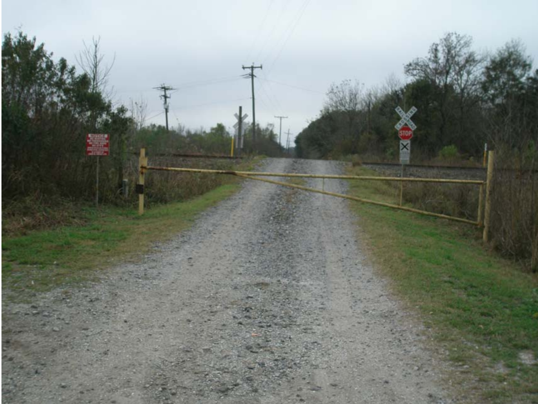
Photo 4: Gated main entrance of the BLP site. December 13, 2007.
