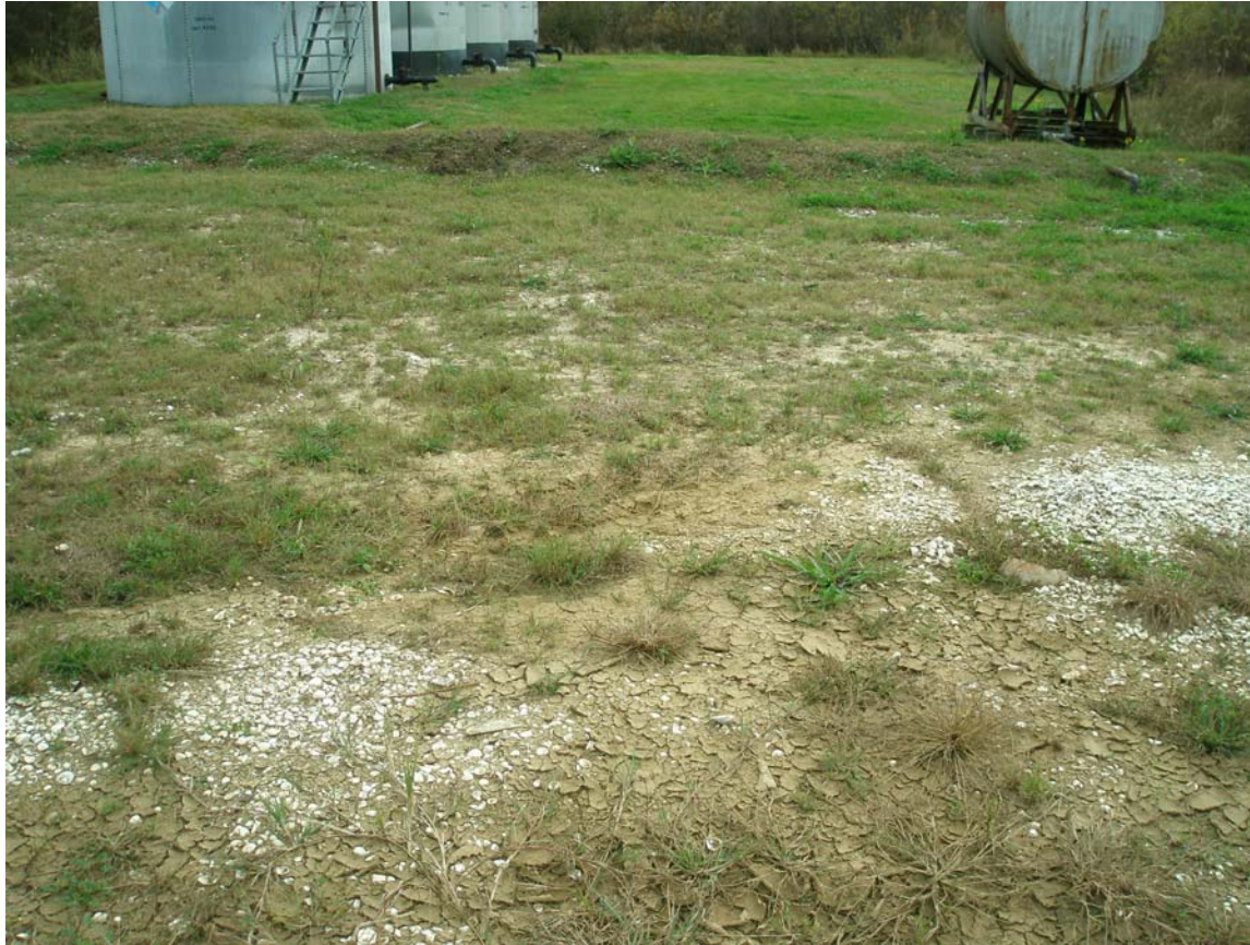
Photo 2: Location of excavation and remediation in area 2. December 13, 2007.
