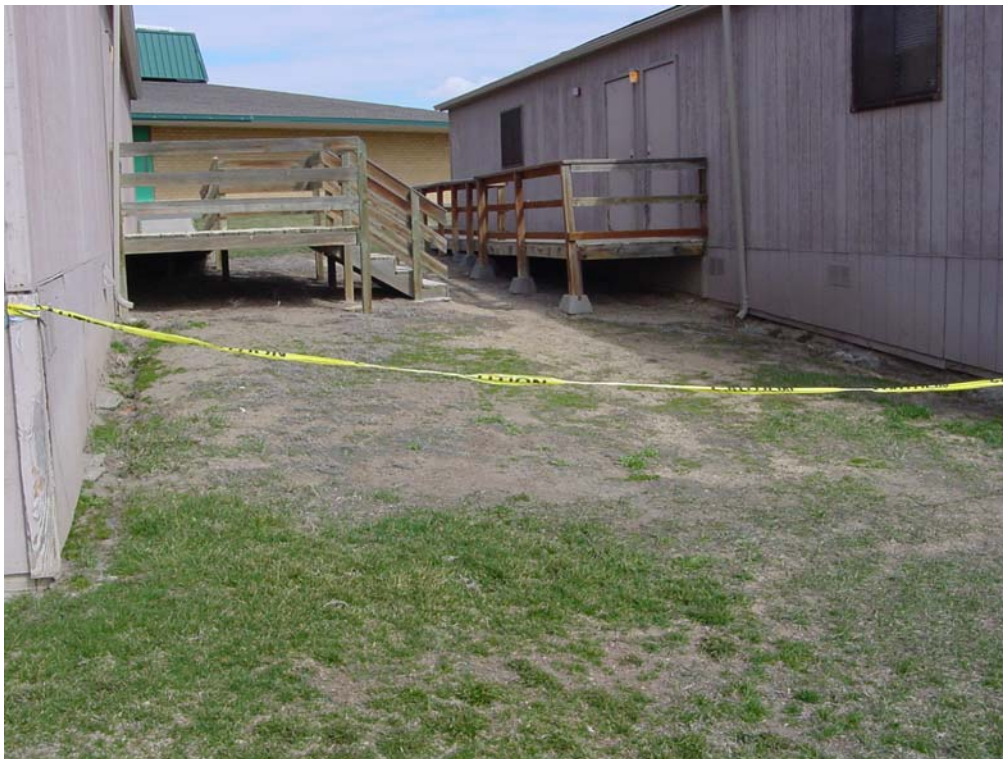
Figure 3. Portable classrooms, Apple Valley Elementary School.
