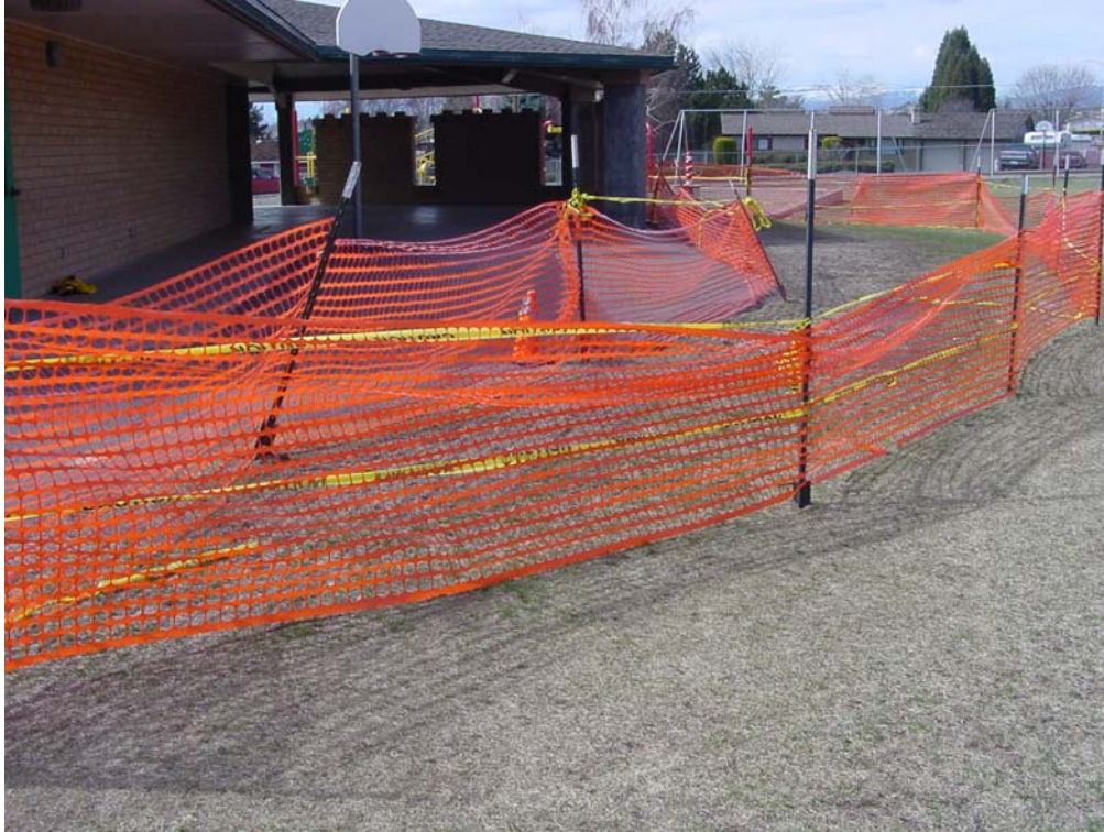
Figure 2. Fenced area of exposed soil, Apple Valley Elementary School.
