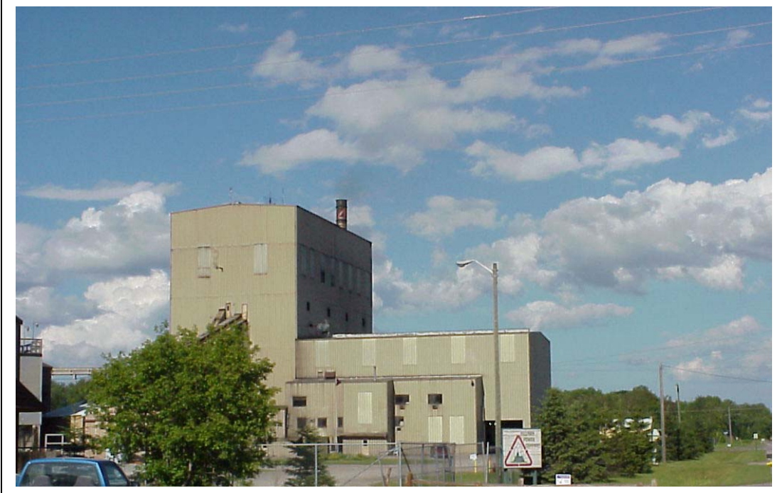
Figure 2a. West view of Hillman Power Company (looking east), village of Hillman, Montmorency County, Michigan.
