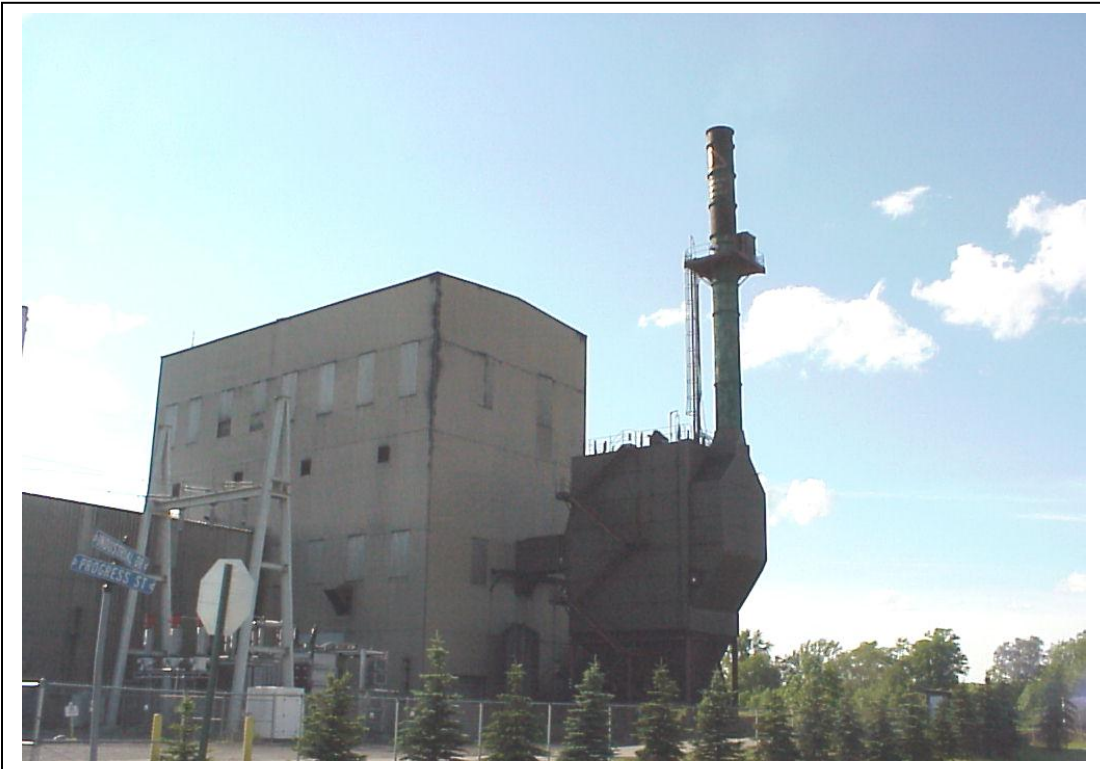
Figure 2b. East view of Hillman Power Company (looking northwest), village of Hillman, Montmorency County, Michigan.
