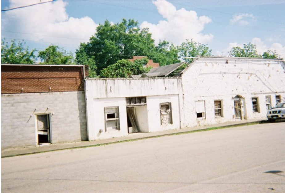
Figure 2. Photo of Side Entrance of Former Cardwell Hospital in Stella, MO.
