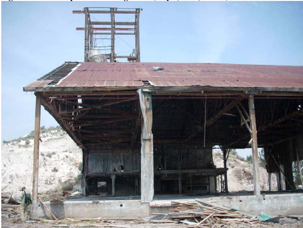
Figure 2. Old mine process building onsite (July 2, 2008; EHAP)
