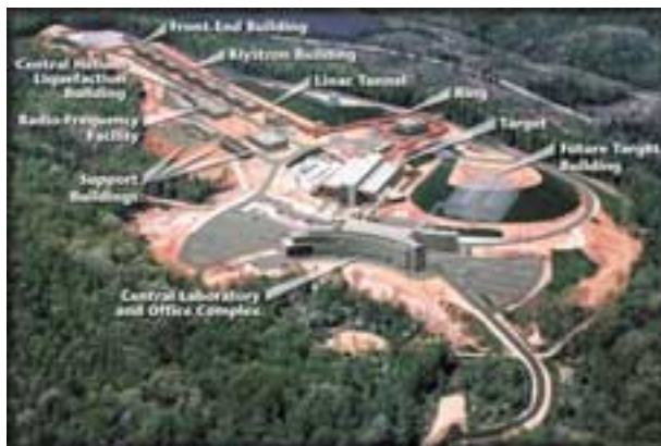
Artist's conception of the Spallation Neutron Source overlaid on the actual construction site in Oak Ridge, TN.
