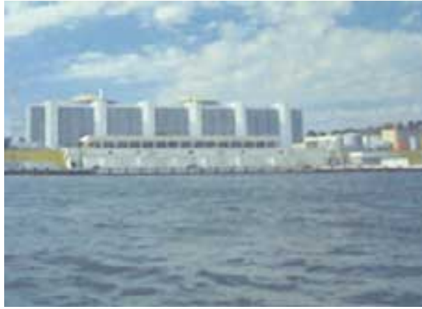
Calvert Cliffs is the first US Nuclear Plant to receive a renewed license from the Nuclear Regulatory Commission. The renewal will allow the plant to continue producing electricity for an additional 20 years.
