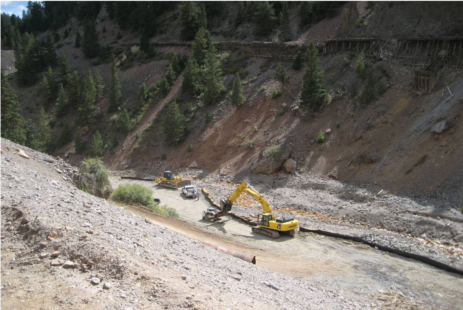
Photo 5: EPA Emergency Response Contractors contouring West Willow Creek Bed (South of NT-CWR Site, Historic Ore Cart Track upper)
