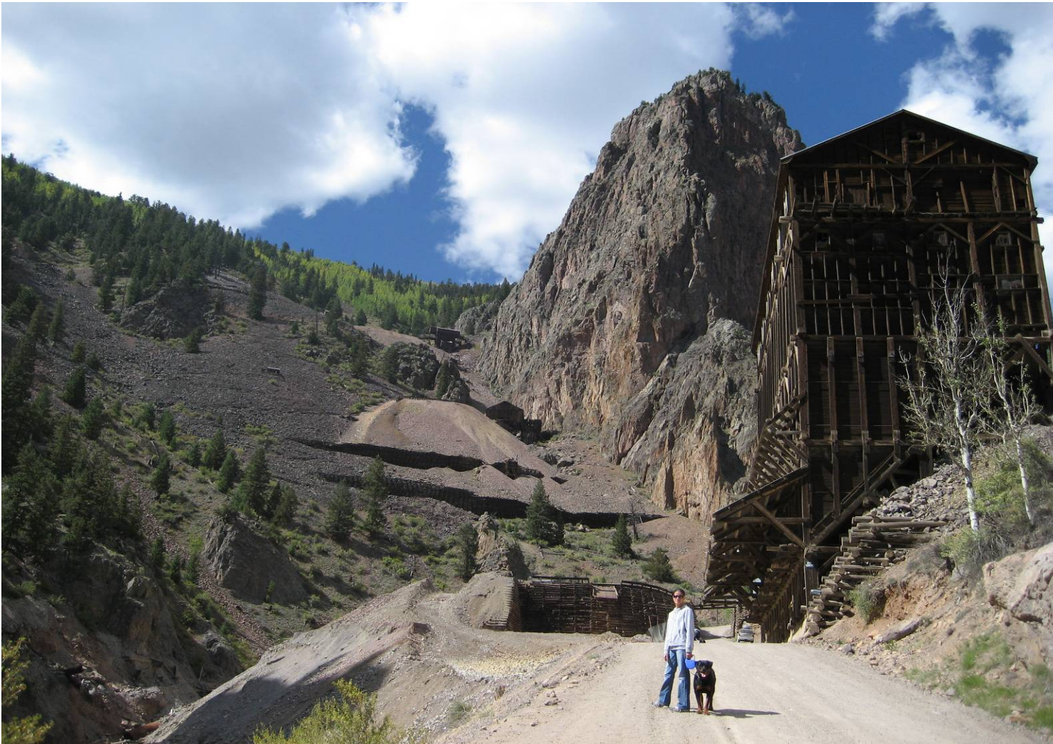
Photo 2: Just south of site at road level (historic loading bin on right, CWR pile and cribbing lower middle, Upper Commodore workings center)
