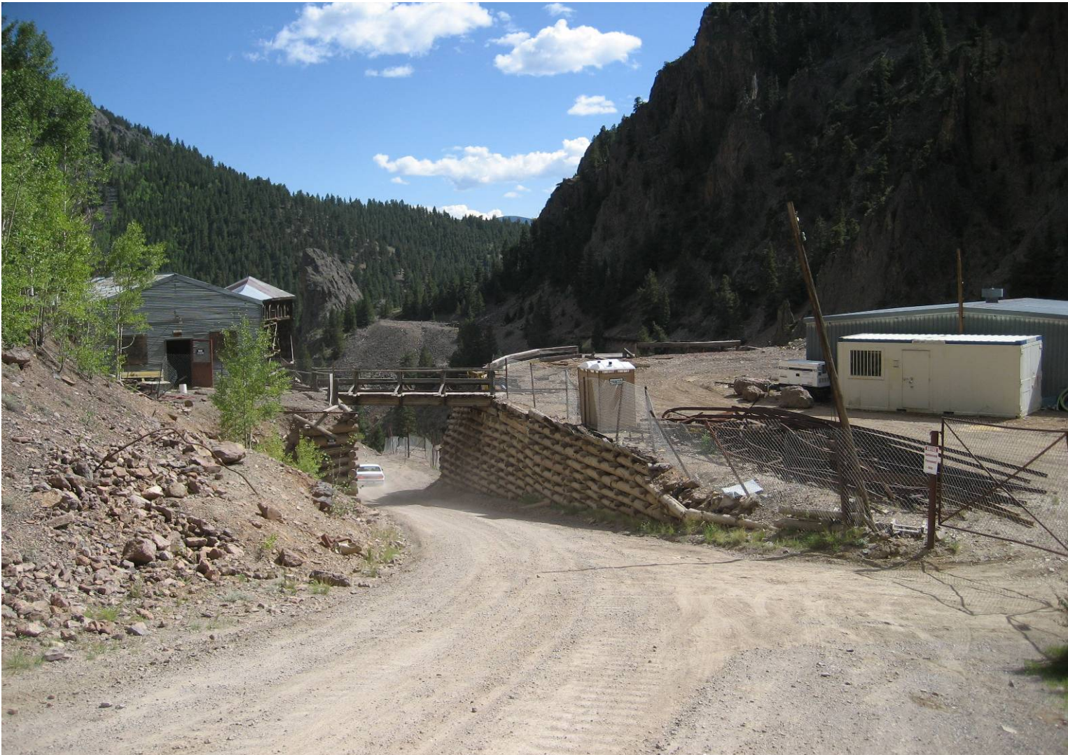
Photo 3: Upper Level of NT-CWR Site looking south (CWR pile on right)
