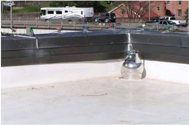
Figure 9. New Castle – Library Monitoring Station, Looking West-southwest
