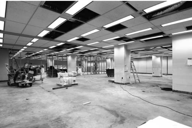
Construction underway in the Madison Building reveals framing for new walls.
