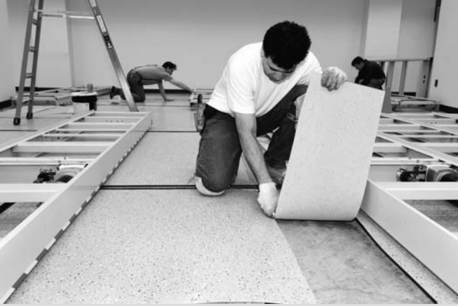
Installation of new flooring
