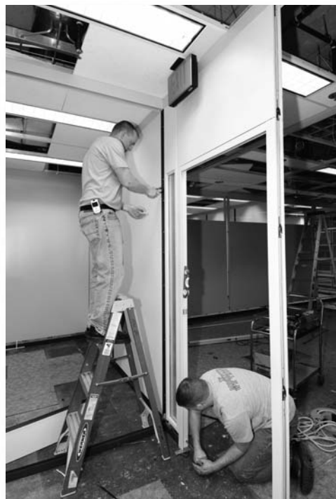
Workers install demountable walls.
