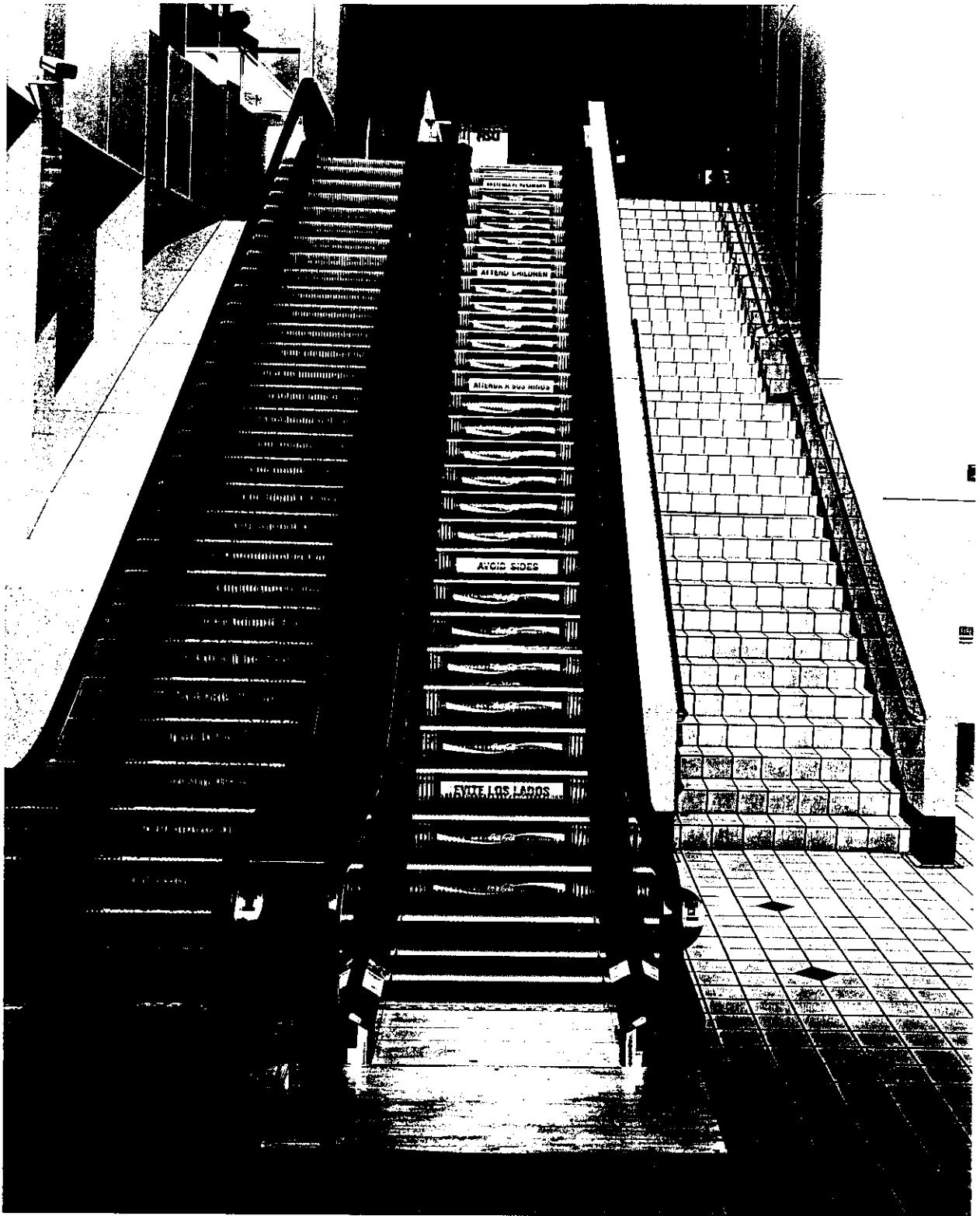
Dallas / Forth Worth International Airport, Dallas, Texas Advertising Signage with Safety Messages every sixth step
