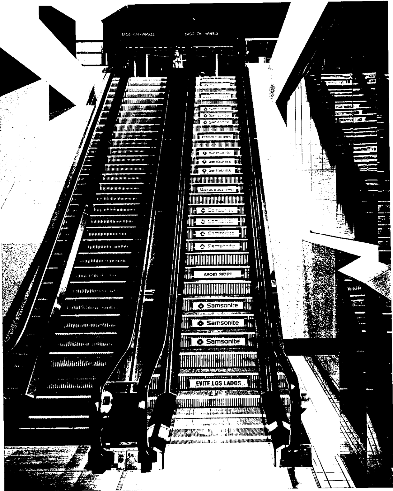
Dallas / Forth Worth International Airport, Dallas, Texas Advertising Signage with Safety Messages every sixth step (blank steps for emphasis) INSTALLED: MAY 1995
