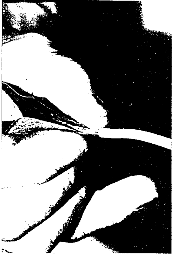
39. THE ALUMINUM WIRE IS ABRADED UNDER THE COATING OF OXIDE INHIBITOR, using, for instance, #220 grit automotive wet-dry finishing sandpaper. This is an important step. Abrasion disrupts and removes much of the insulating oxide, and the inhibitor film prevents fresh oxide formation on the bare aluminum.
