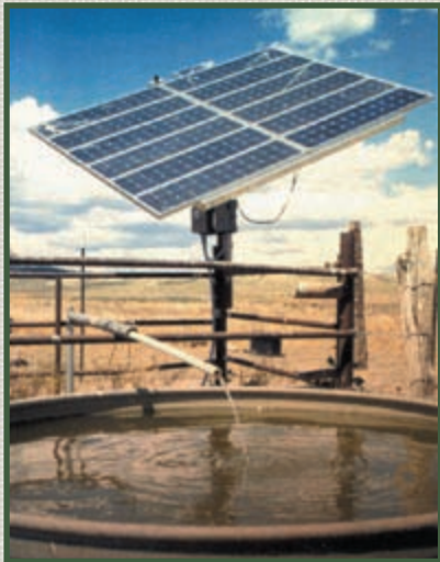
Ute Mountain Indian Reservation solar water pumping
