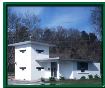
The Oak Ridge Turnpike Checking Station contains World War II-era furnishings.
