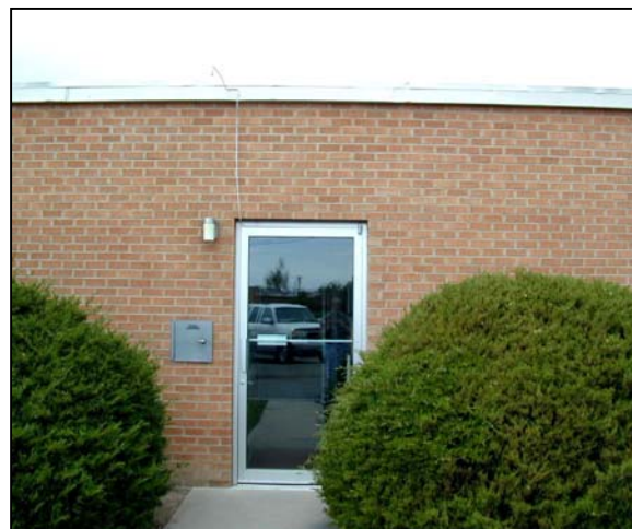
Site Photo: VOC inlet, to west
