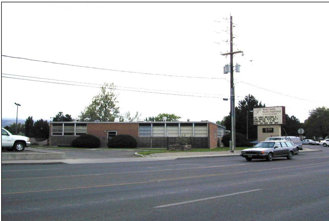
Site Photo: Looking Southwest
