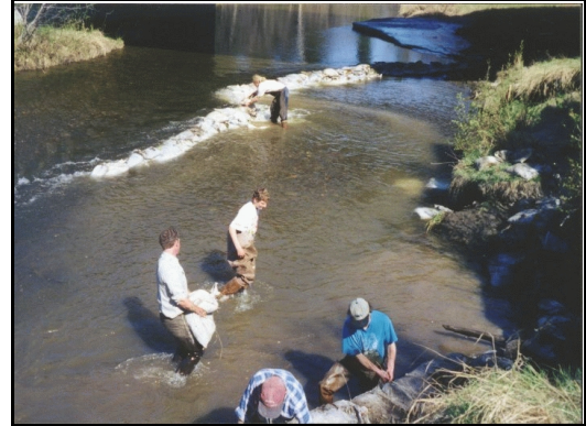
Volunteers removing sandbags
