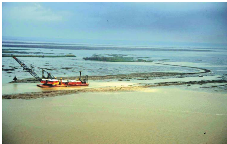
A bucket dredge is shown removing sediment from a shoaled-in channel in order to help reestablish water and sediment flow within the Atchafalaya Delta.
