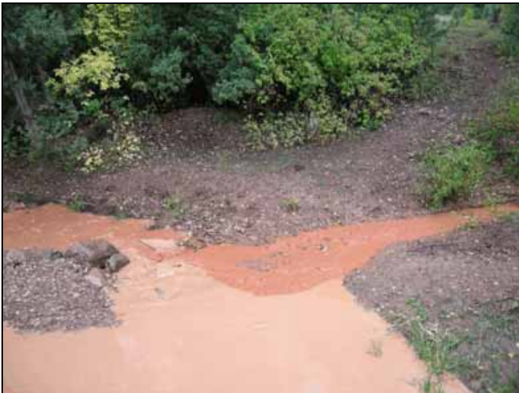
Plate 1.2 Roads, unstable slopes, and other nonpoint sources of pollution have been observed to increase sedimentation problems from stormwater runoff at many locations throughout the Diamond Fork Watershed (top and bottom photos were taken in areas of recent construction in the upper Diamond Fork above Three Forks portion of the watershed).
