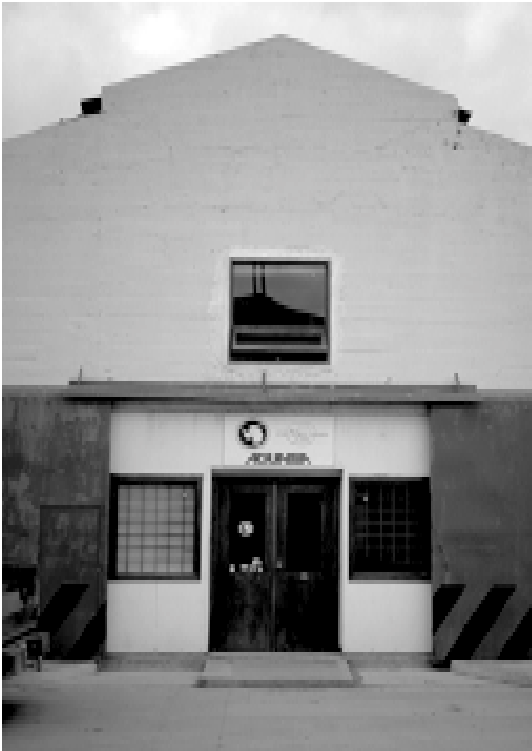
Figure 3-2: Punta Arenas warehouse. (photo by Tim Cully)
