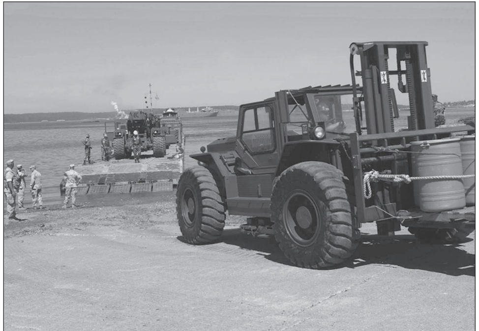
Figure 3: Navy Forces Use a Barge to Move Construction Vehicles During a Joint Logistics-Over-the-Shore Exercise at Naval Magazine, in Indian Island, Washington
