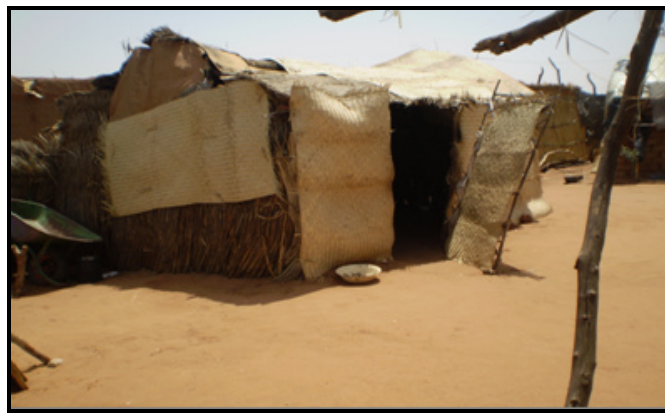
3.1b: Typical house construction in Otash Camp
