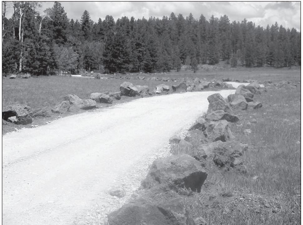
Figure 4: Barrier Rocks Placed along Dixie National Forest Roadway to Prevent Off-road Vehicle Use
