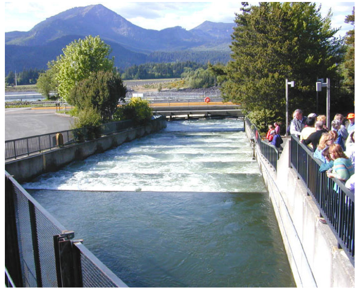
One of several fish ladders located at Bonneville Dam on the Columbia River, looking down the approximately 60 1-foot steps of the "ladder." Photo Credit: Eric Guinther.
