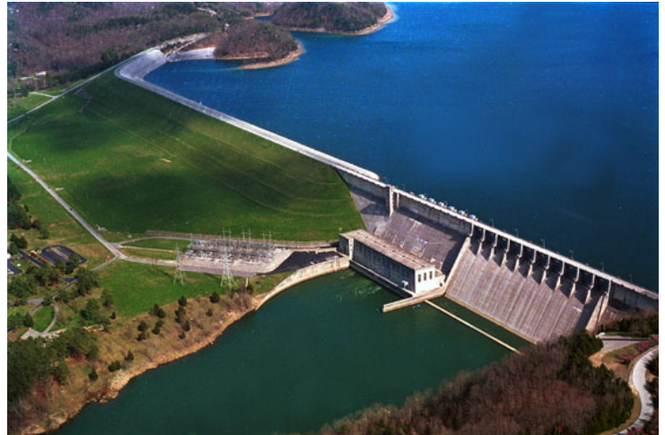
Wolf Creek Dam and hydroelectric power plant. Photo Credit: U.S. Army Corps of Engineers Nashville District.
