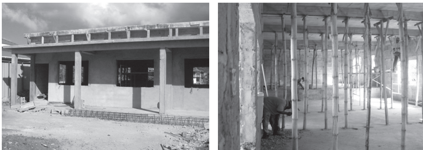
Figure 5: USAID-Funded School Repair in Grenada
