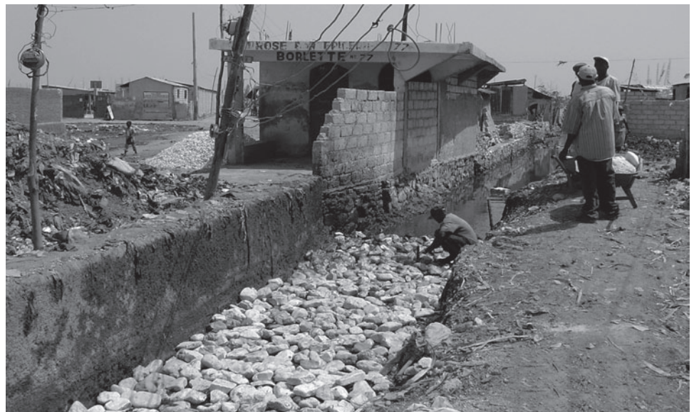
Figure 4: USAID-Supported Drainage Canal Cleanup in Haiti
