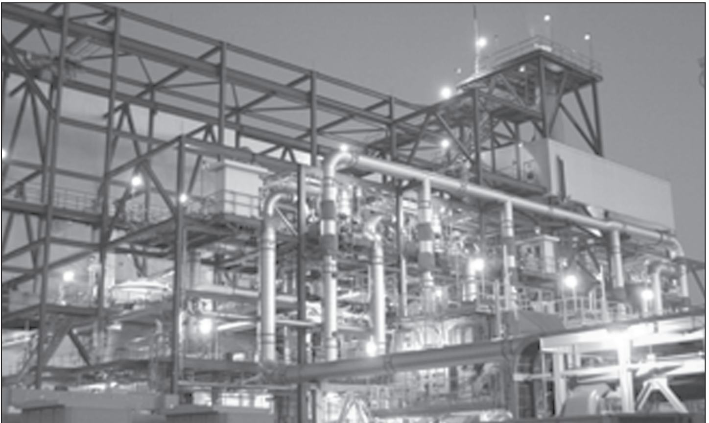
Figure 2: Umatilla Chemical Agent Disposal Facility, Umatilla Chemical Depot, Oregon
