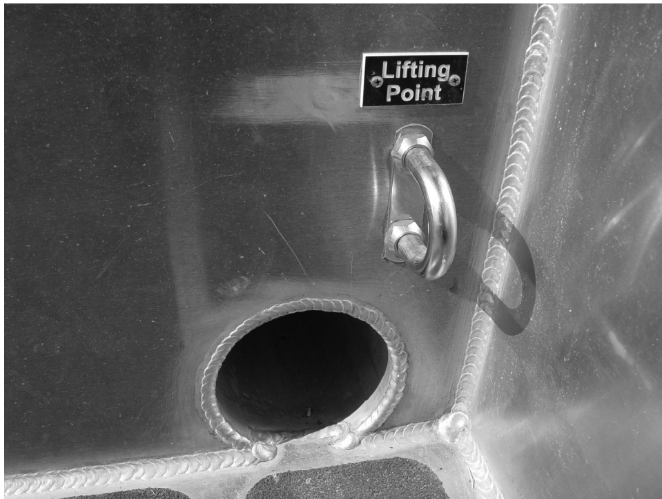
Figure 2-23 Lifting Eye
