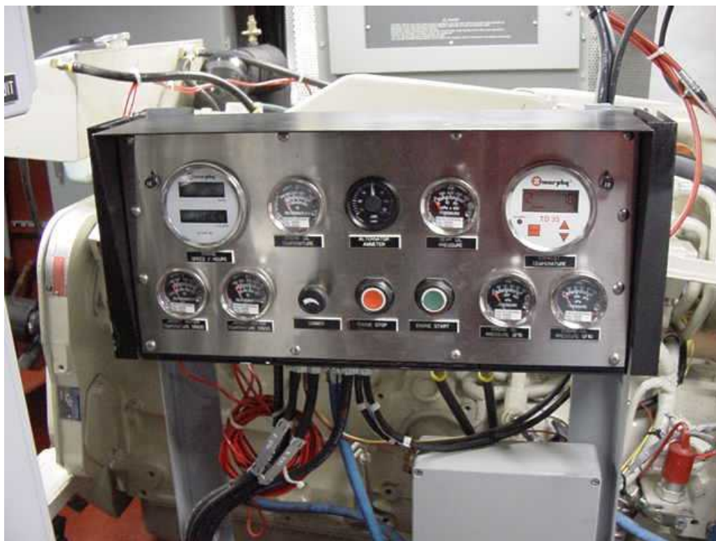
Figure 3-17 Engine Starting System
