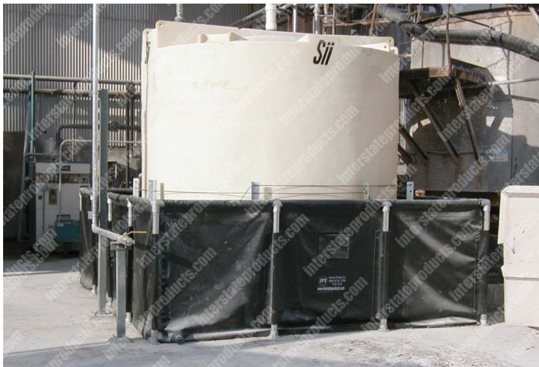
Figure 3.5: Example commercial secondary containment system which would be attached to the interior side of the drywall walls of the IPND structure inside the existing MINOS Service Building.
