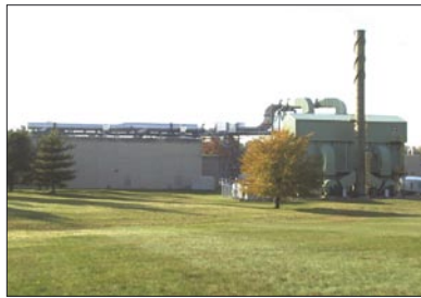
Large Fire Laboratory (left) and Flue Gas Cleaning System (right).
