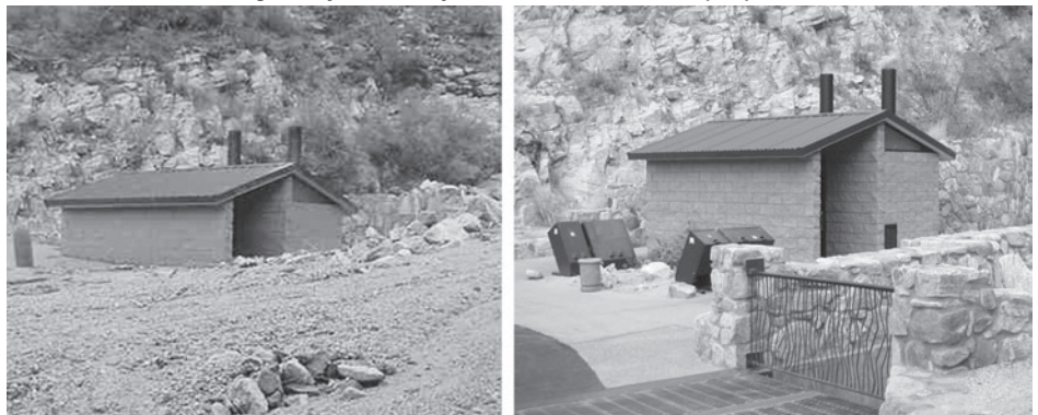
Forest Service Building Partly Buried by Postfire Flood Debris (left) and Restored Later
