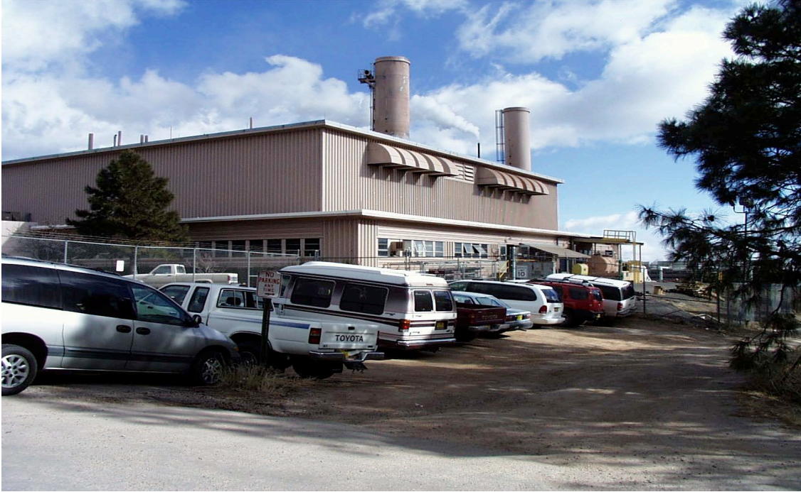
Figure 2-1. Main Steam Plant at LANL TA-3.
