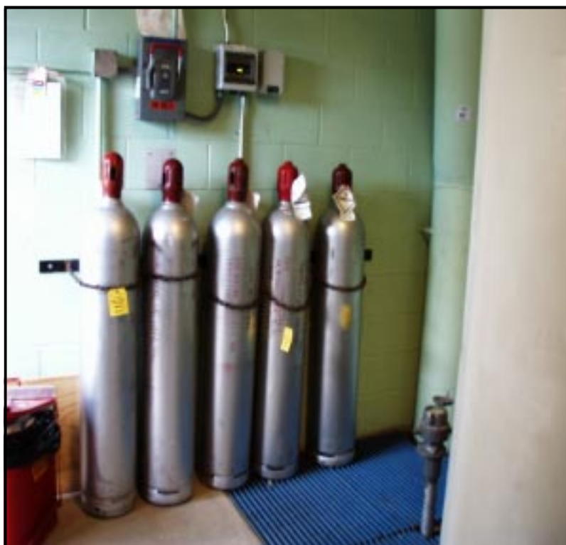
Fig. 7-4. Chlorine gas cylinders.
