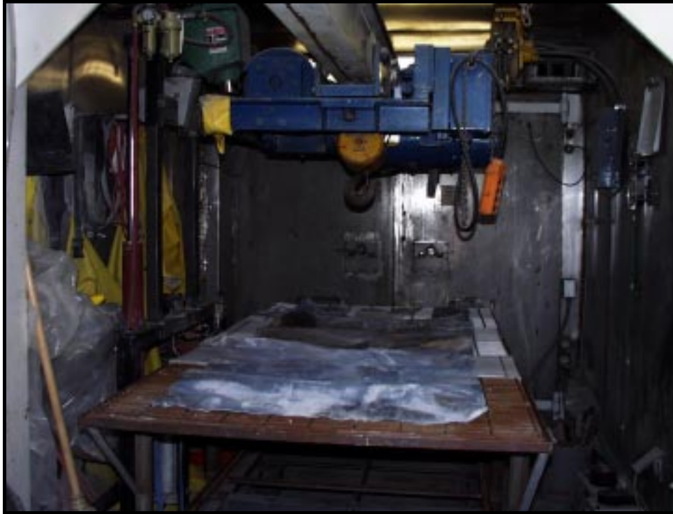
Fig. 7-5. Lead decontamination site.
