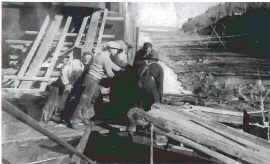
Unloading the dredge pontoons at Coal Creek. The man facing the camera (in the overalls) is Frank Slaven. His roadhouse is visible on the high bank at the upper right. Note the tripods that supported a telephone line which allowed the crew on the beach to communicate with the camp approximately 7 miles up Coal Creek. George Beck Collection, photograph courtesy of Max Beck.
