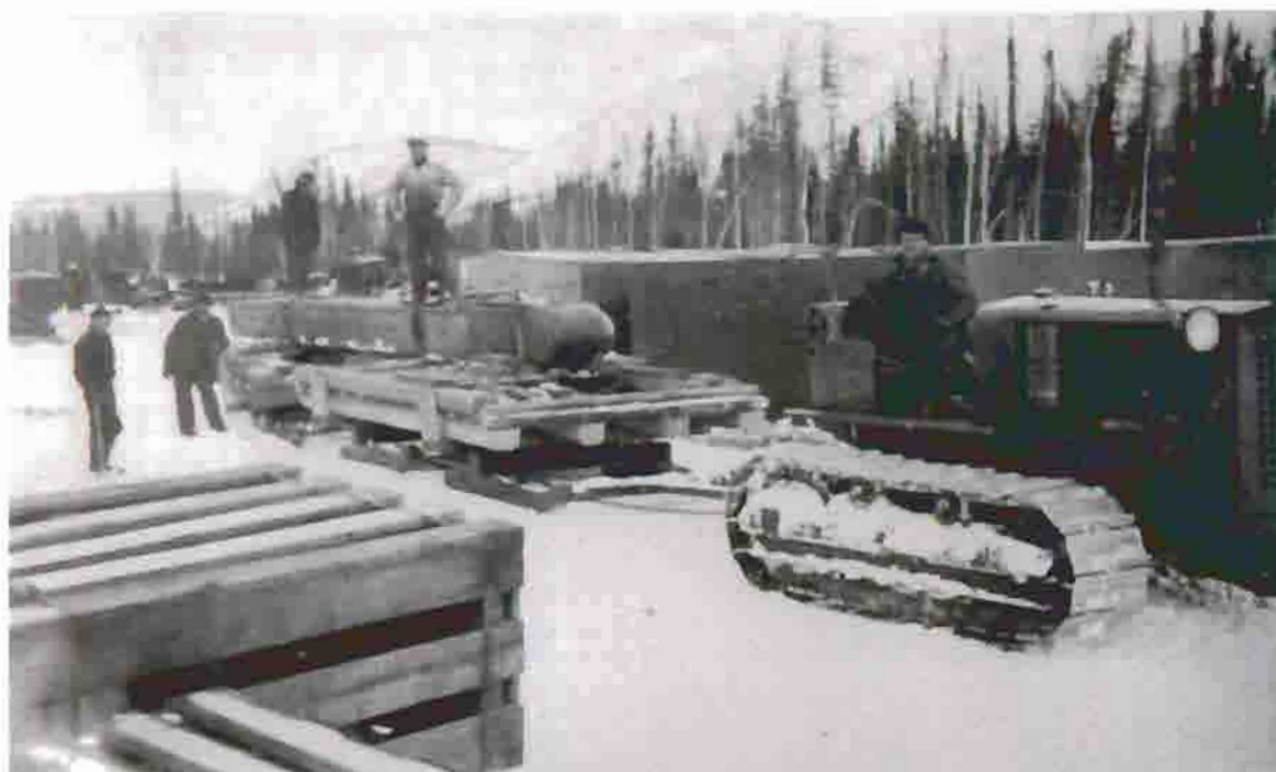
Hauling dredge parts from the Yukon River to Camp No. 1 where the dredge was assembled. George Beck is driving the tractor pulling the spud. The sled on which the spud is lying is currently located near the Coal Creek airstrip. George Beck Collection, photograph courtesy of Max Beck.
