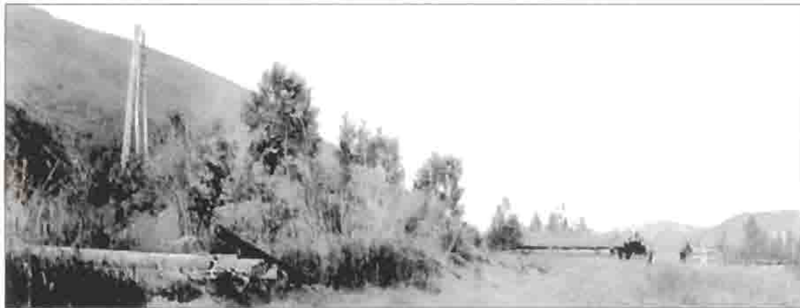
Early mining camp on Coal Creek. This is likely Frank Slaven's claims and operation. Note the gin pole on the left for hauling paydirt out of the ground and the two cabins on the right. Frank Slaven Collection, courtesy of Sherrie Harrison.
