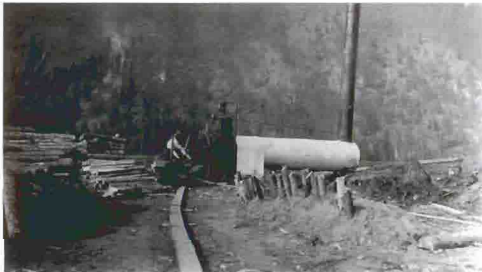
Boiler on Coal Creek with cordwood (1935). Gold Placers, Inc. used steam thawing for the first season or two of work on Coal Creek. After that, they pioneered the use of cold water thawing, thus saving a considerable amount of labor and money spent previously to cut cordwood and fire the boiler. The "scar" on the hill in the upper left of the photo is the end of the Coal Creek Ditch. This boiler is located near the machine shop and parts warehouse near the confluence of Cheese Creek and Coal Creek. Frank Slaven Collection, photo courtesy of Sherrie Harrison.
