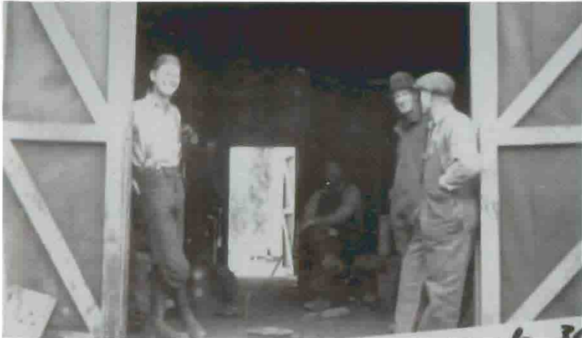
This is the only known photograph of the machine shop showing the crew and the interior of the shop. It was taken in the late 1930s. (NPS Collection, photo by Bill Lemm).
