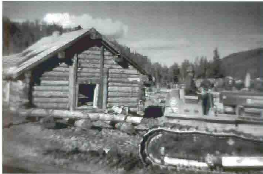
The Gold Placers Inc. TD-24 moving a cabin. Note the skid logs placed under the cabin to slide it from place to place. Harry Gingrich is operating the tractor. Dale and Karen Patty Collection, photograph courtesy of Dale and Karen Patty.
