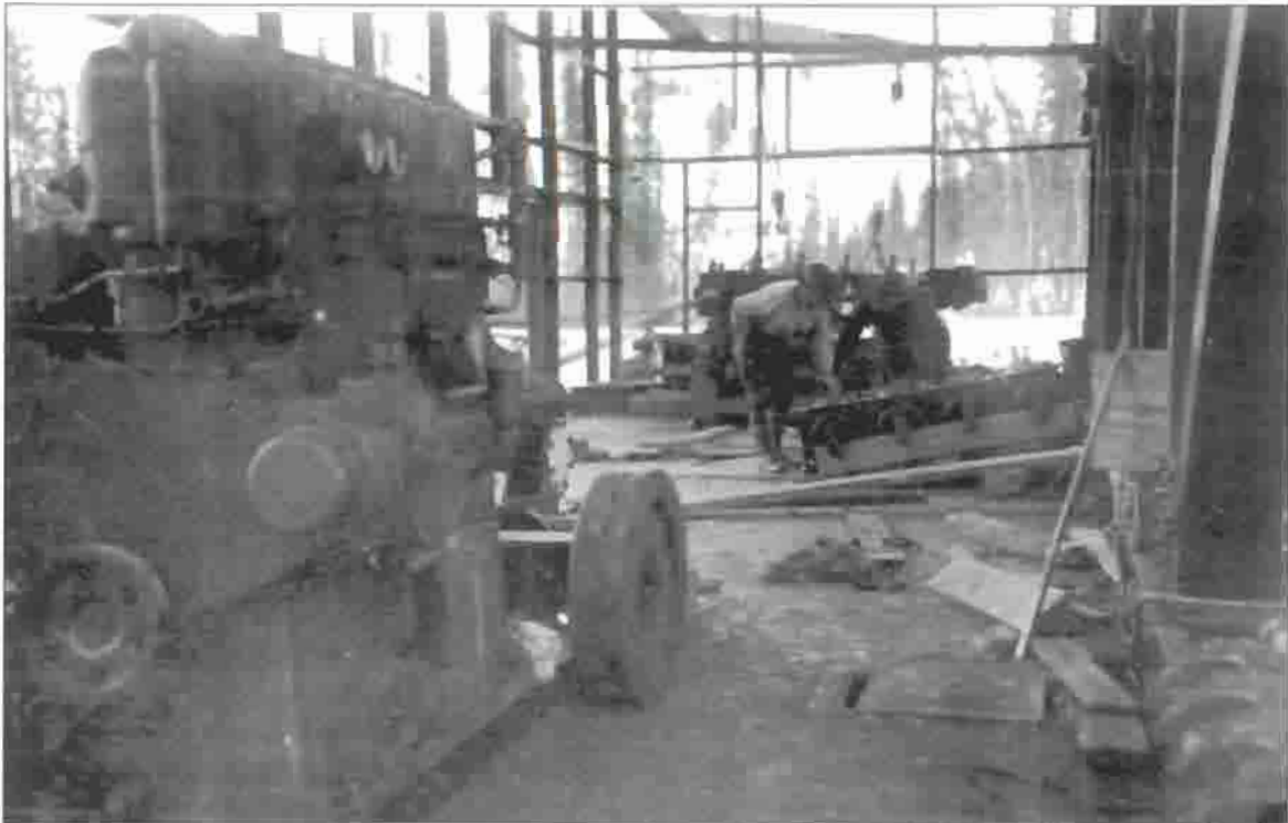
Atlas diesel engines under construction on the main deck. The engine to the left ran the pumps while the engine in the background ran the bucket line, screen, winches and stacker. George Beck Collection, photograph courtesy of Max Beck.
