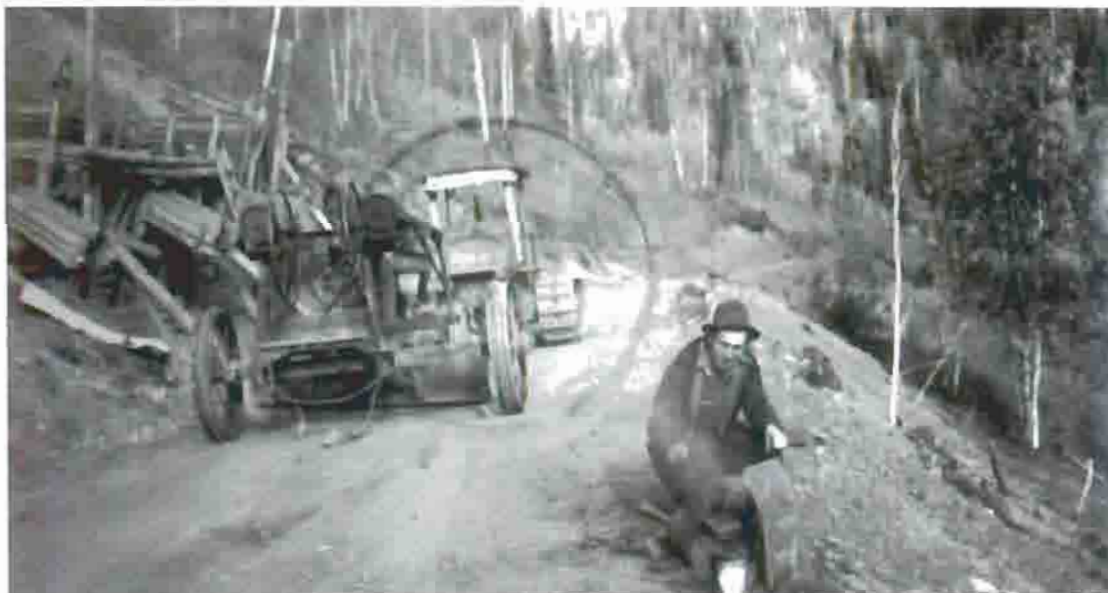
Alaska Road Commission (ARC) grader at work on the Coal Creek Road approximately 1½ miles above the Yukon River. NPS Photo, Bill Lemm Collection.
