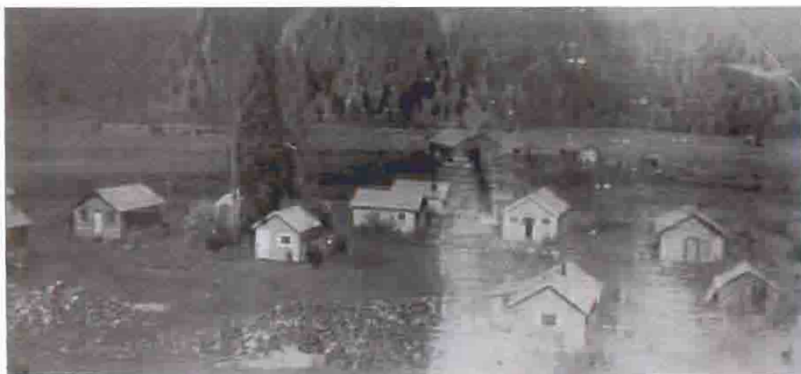
Camp #1 located across from Cheese Creek. The machine shop is the large building in the center rear of the photograph. The tractor garage and parts warehouse is the second building to the right (with the large white garage doors). The blacksmith shop sits between the two. The dredge is visible in the far right near the base of the hill. (Photo courtesy of Glen Franklin).
