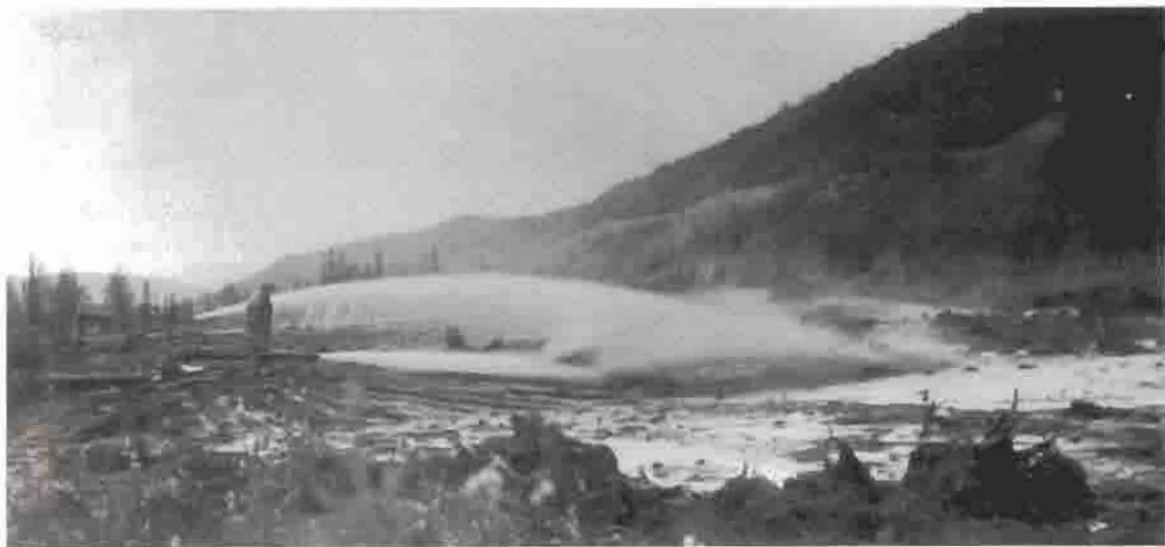
Using a hydraulic giant to thaw and strip away the "muck" that covers the alluvial gravel on Coal Creek. Everett Hamman Collection, University of Alaska-Fairbanks.
