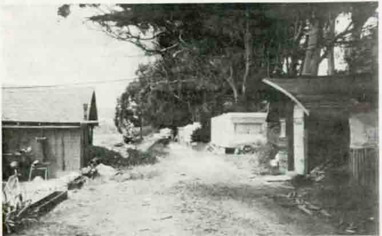
Figure 36 - Looking north from parking lot, 1986. From Appraisal .
