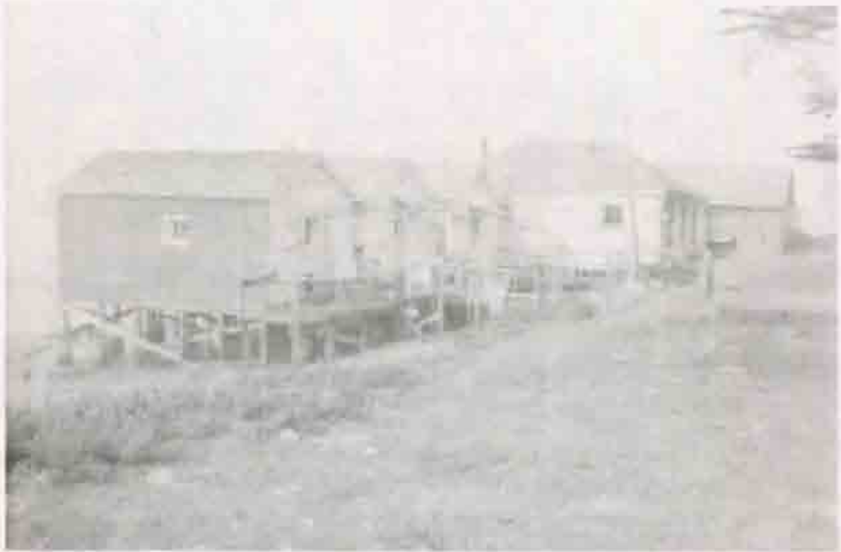
Figure 21 - North complex from railroad grade, view to north. Left to right: structures 11, 13, 15, 17, 18.
