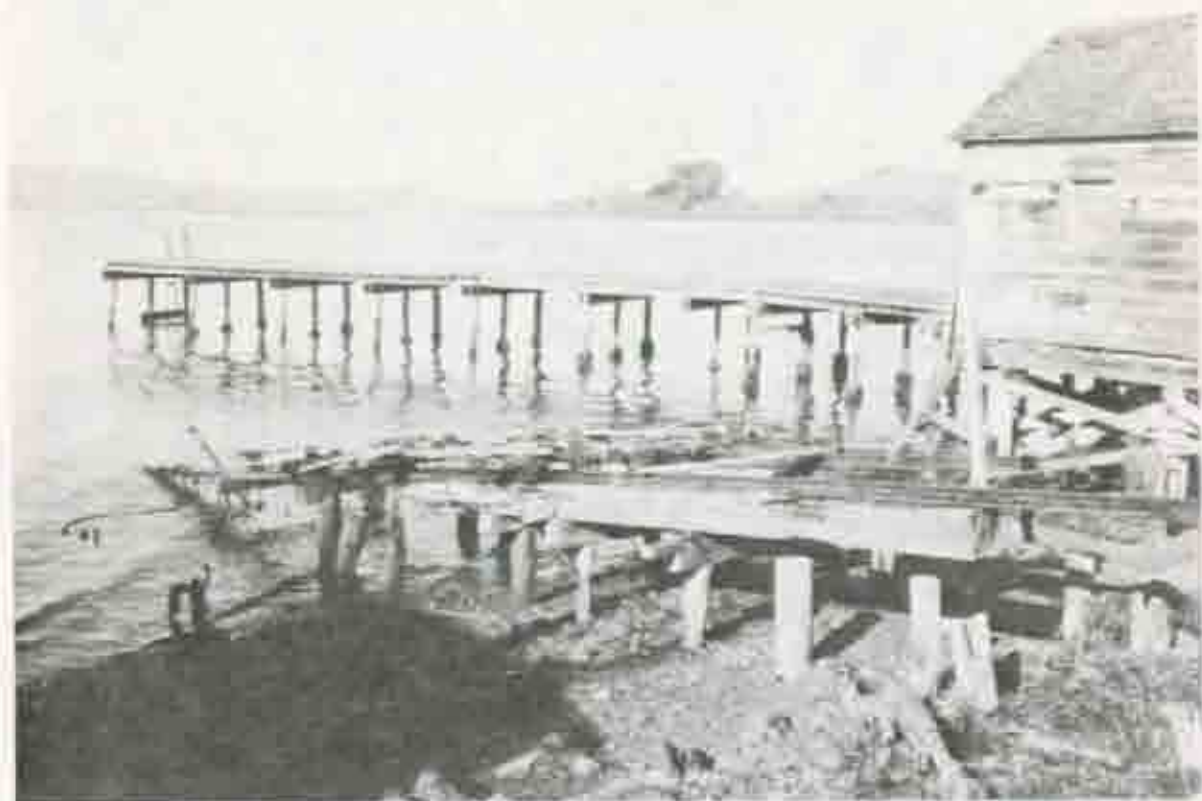
Figure 10 - Structure 6, boat ways, view to northwest, wharf behind.
