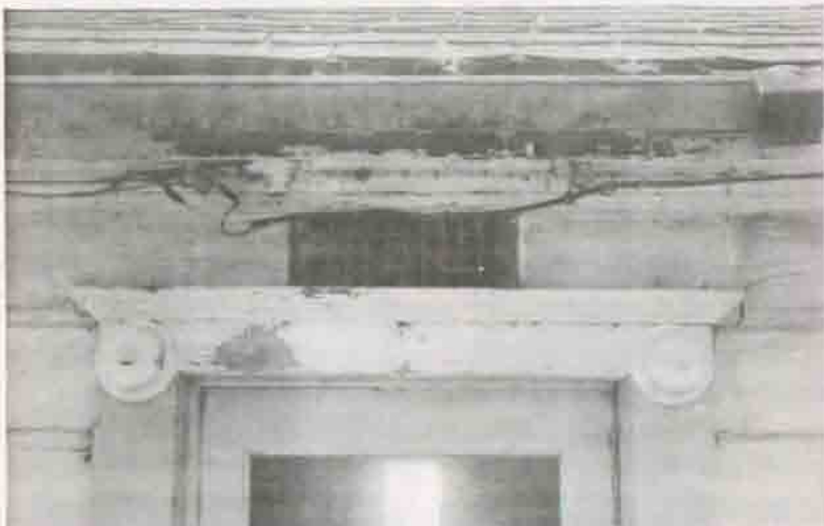
Figure 27 - Structure 17, Spiegel cabin, decoration over front (east) door.
