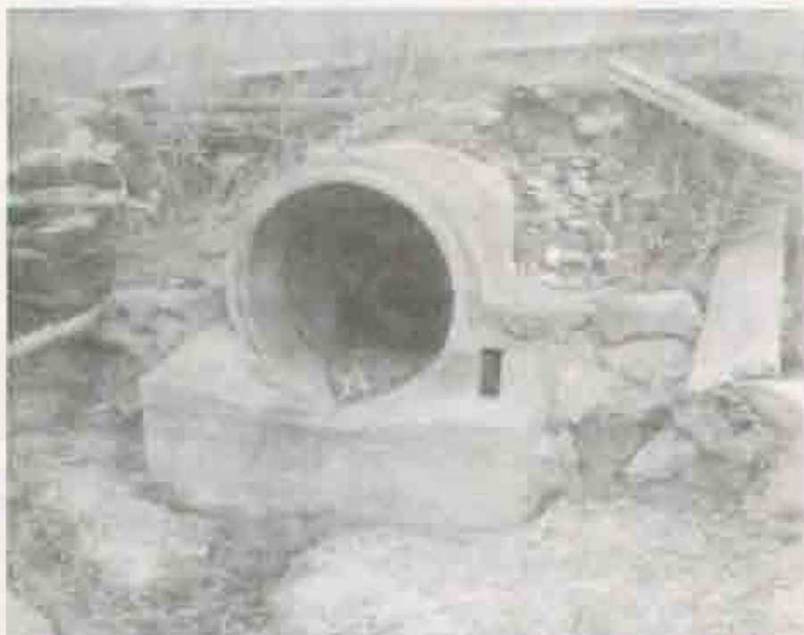
Figure 19 - Culvert directly north of Structure 10. View to east.
