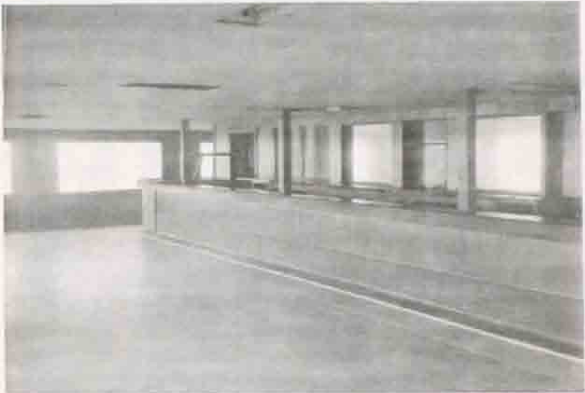
Figure 15 - Structure 9, restaurant, interior. View to west.
