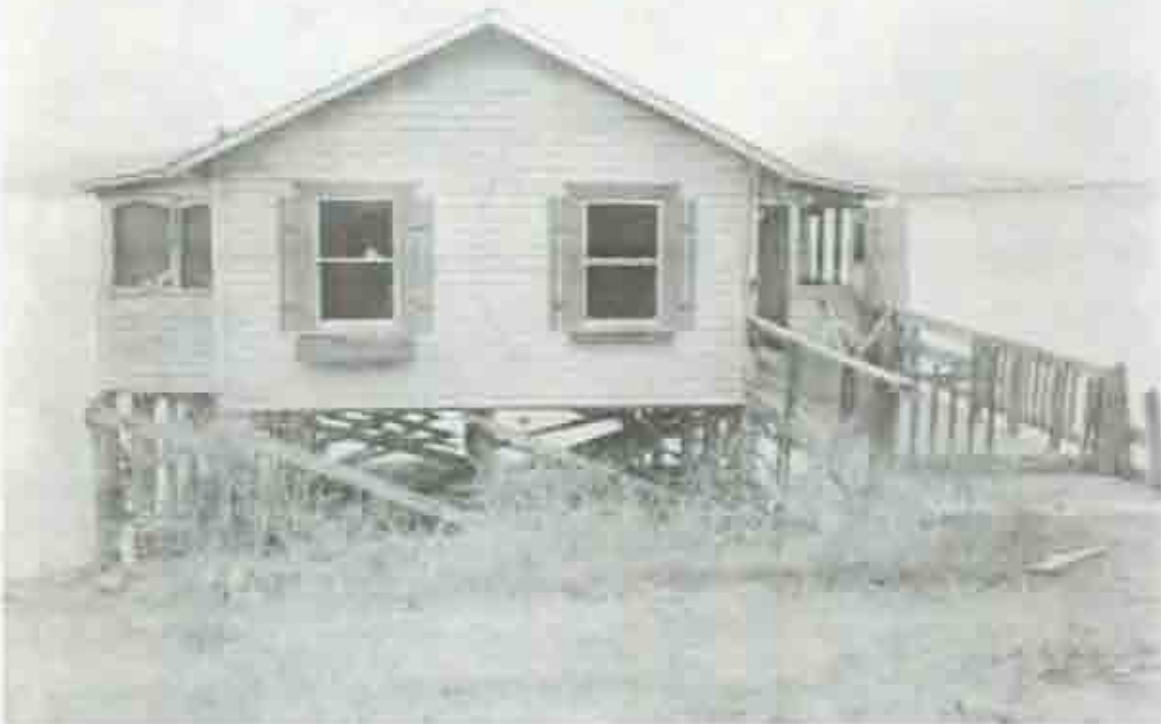
Figure 5 - Structure 3, Lacey cabin, east side.
