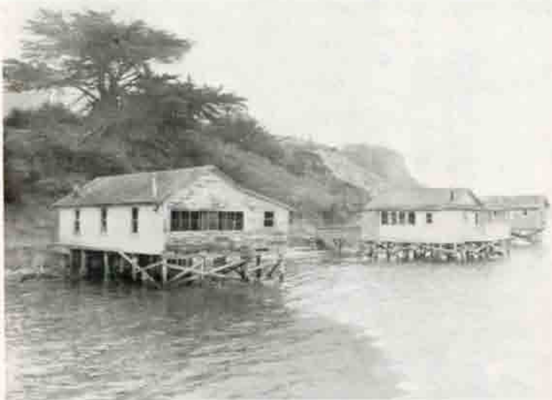
Figure 9 - Structures 5, 3, 2 from wharf, view to southeast.
