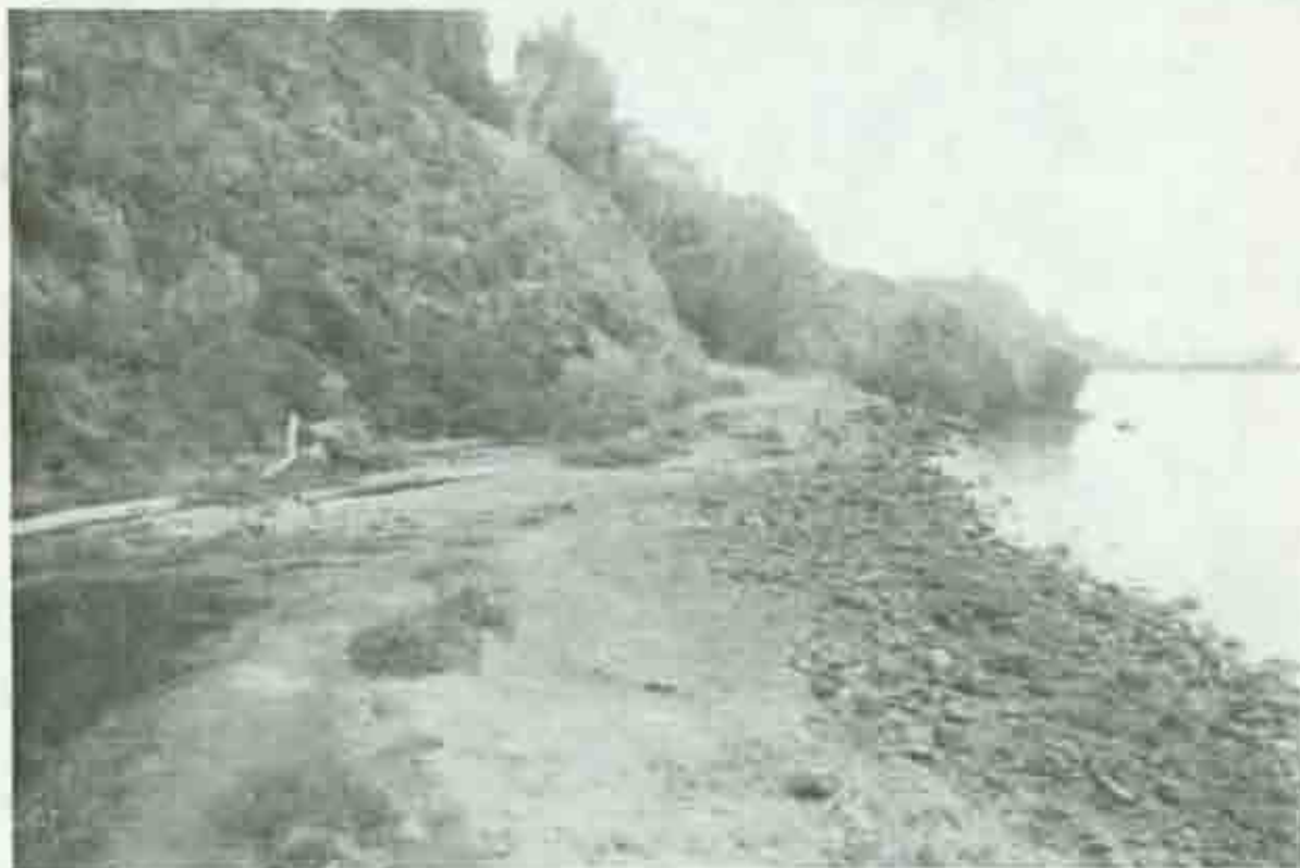
Figure 34 - View to south at south end of property, of railroad grade (CA-MRN-560). Remains of fill in foreground, large cut in center. Nick's Cove in distance.
