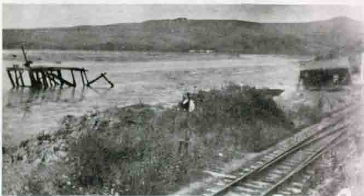
Figure 8 - Earthquake damage, 1906, showing the fallen wharf and depot. No other buildings appear at the water line. T.E.L.H.C.
