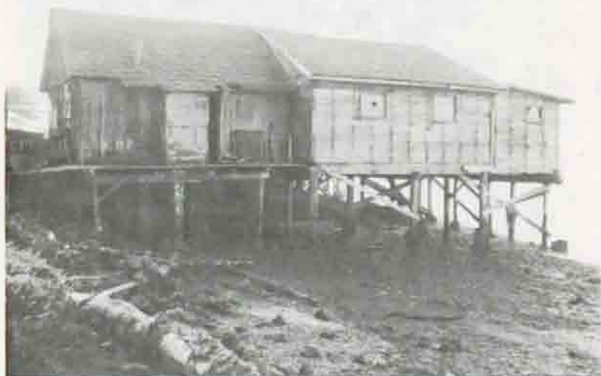
Figure 30 - Structure 18, Price cabin, north side.
