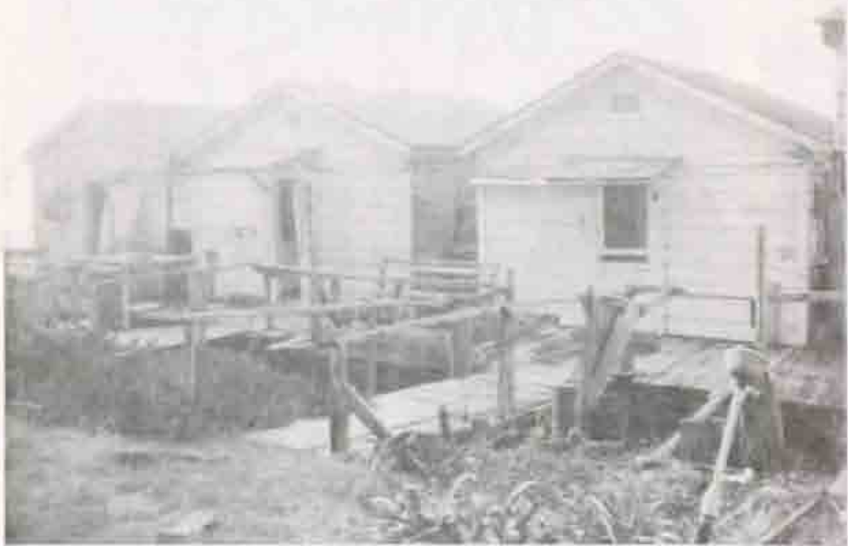
Figure 22 - Structures 11, 13, 15, east sides.
