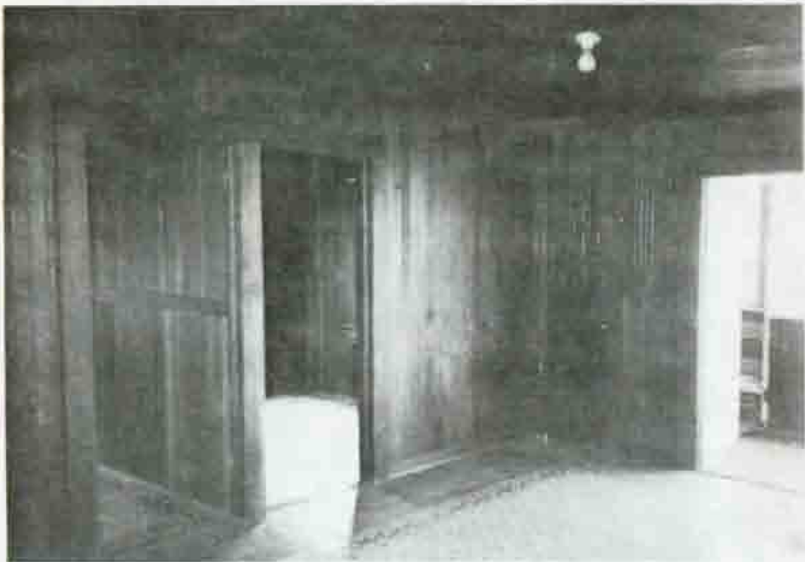
Figure 6 - Structure 3, Lacey cabin, interior view.
