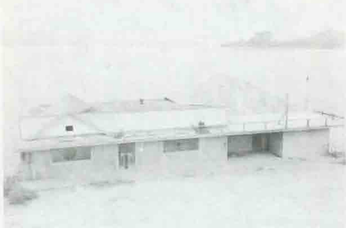
Figure 12 - Structures 9 and 10, restaurant and Jensen house, view to west from hill. Preston Point in distance.
