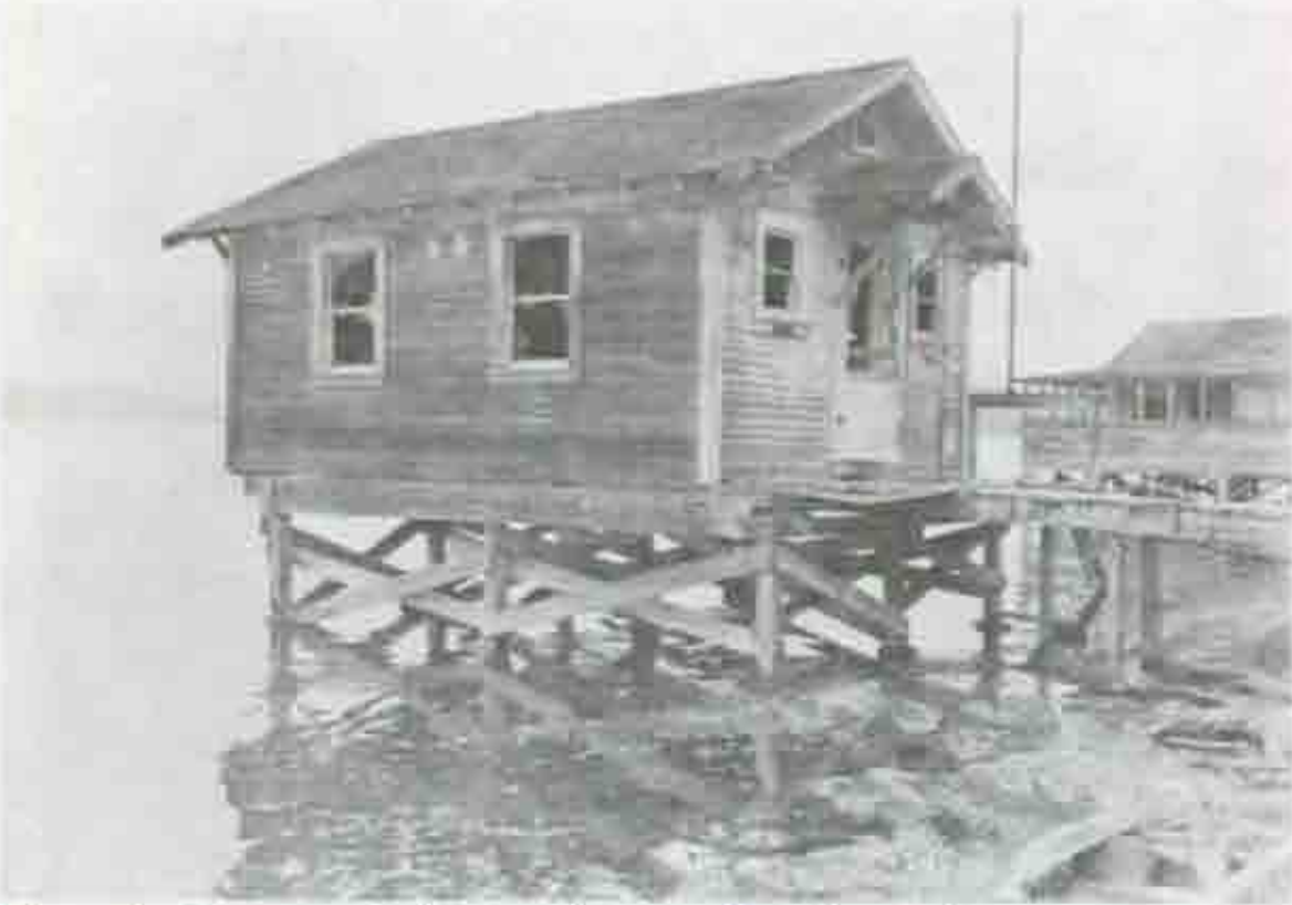
Figure 4 - Structure 2, old shoe shop, south and east sides.
