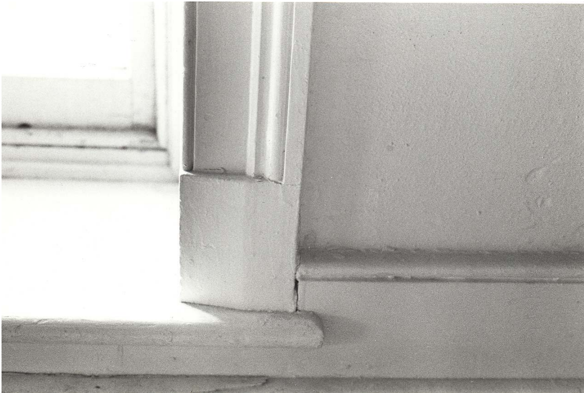
Figure 278. Dwelling interior: detail of elaborate window trim in southwest bedroom (1983).
