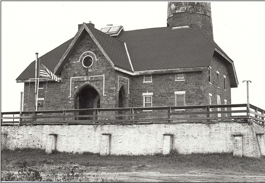
Figure 227. Dwelling exterior: south and east elevations (1982).
