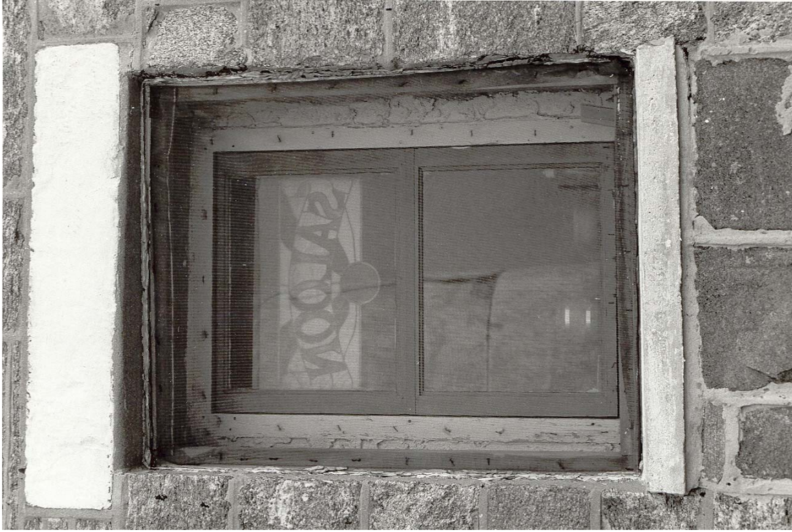
Figure 261. Dwelling exterior: north wall of west apartment, center window (1983).
