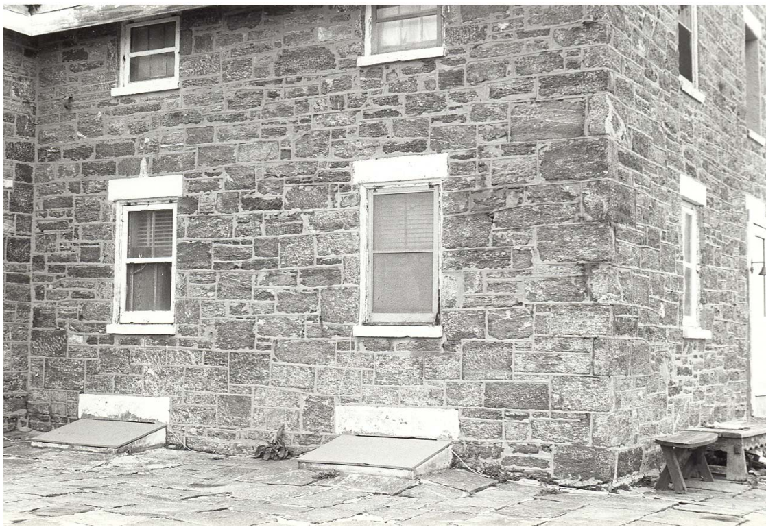
Figure 228. Dwelling exterior: south wall of east apartment, windows (1982).
