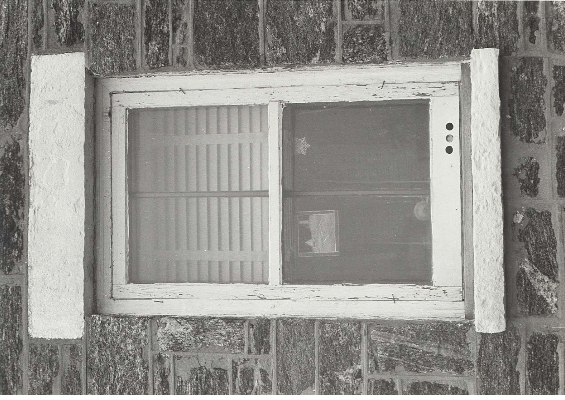
Figure 263. Dwelling exterior: east wall, south window (1982).
