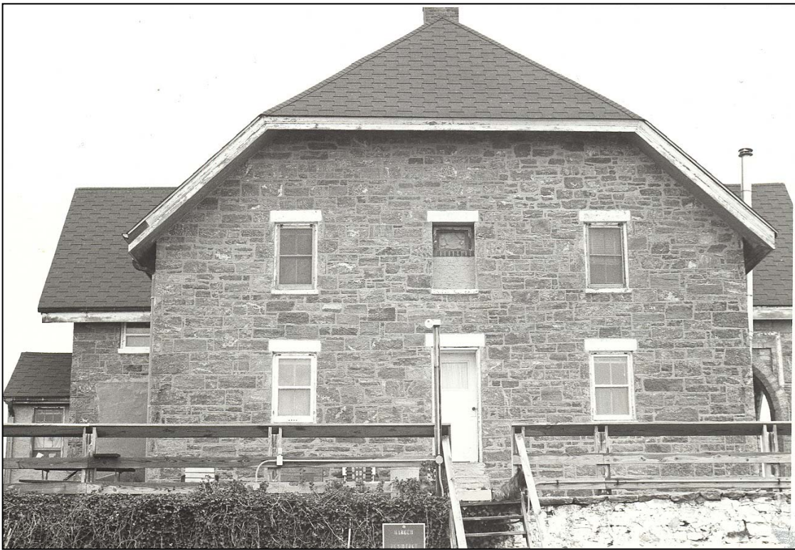
Figure 236. Dwelling exterior: west wall with Type-IV mortar joints (1982).
