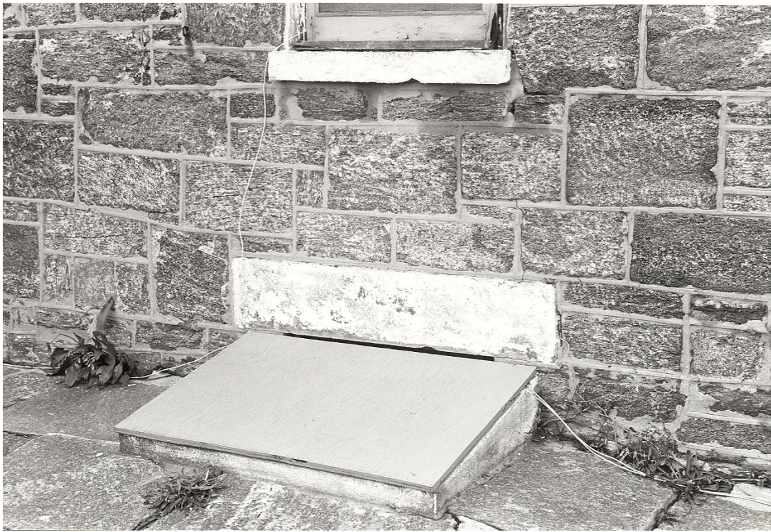
Figure 258. Dwelling exterior: south wall of east apartment, window well (1982).
