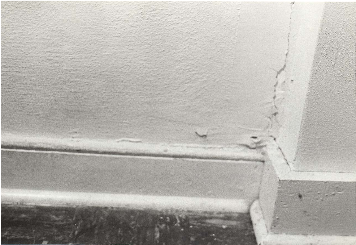
Figure 273. Dwelling interior: Type-III baseboard (1983).
