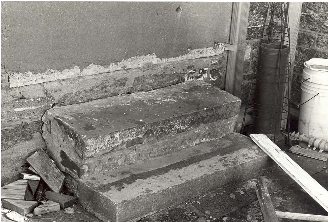
Figure 248. Dwelling exterior: north pavilion, steps for former west doorway (1983).
