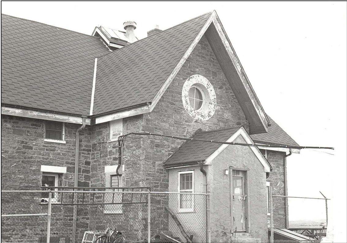
Figure 234. Dwelling exterior: north elevation, pavilion, and vestibule (1982).
