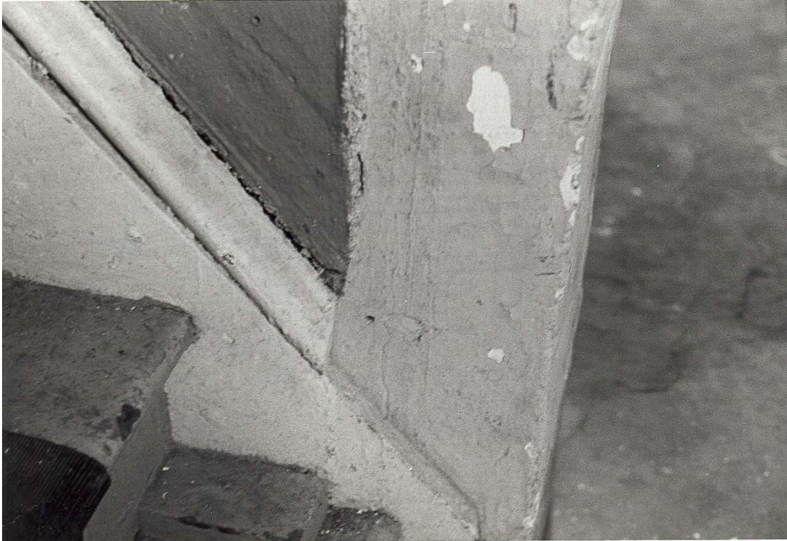
Figure 281. Dwelling interior: detail of cellar stairway (1983).
