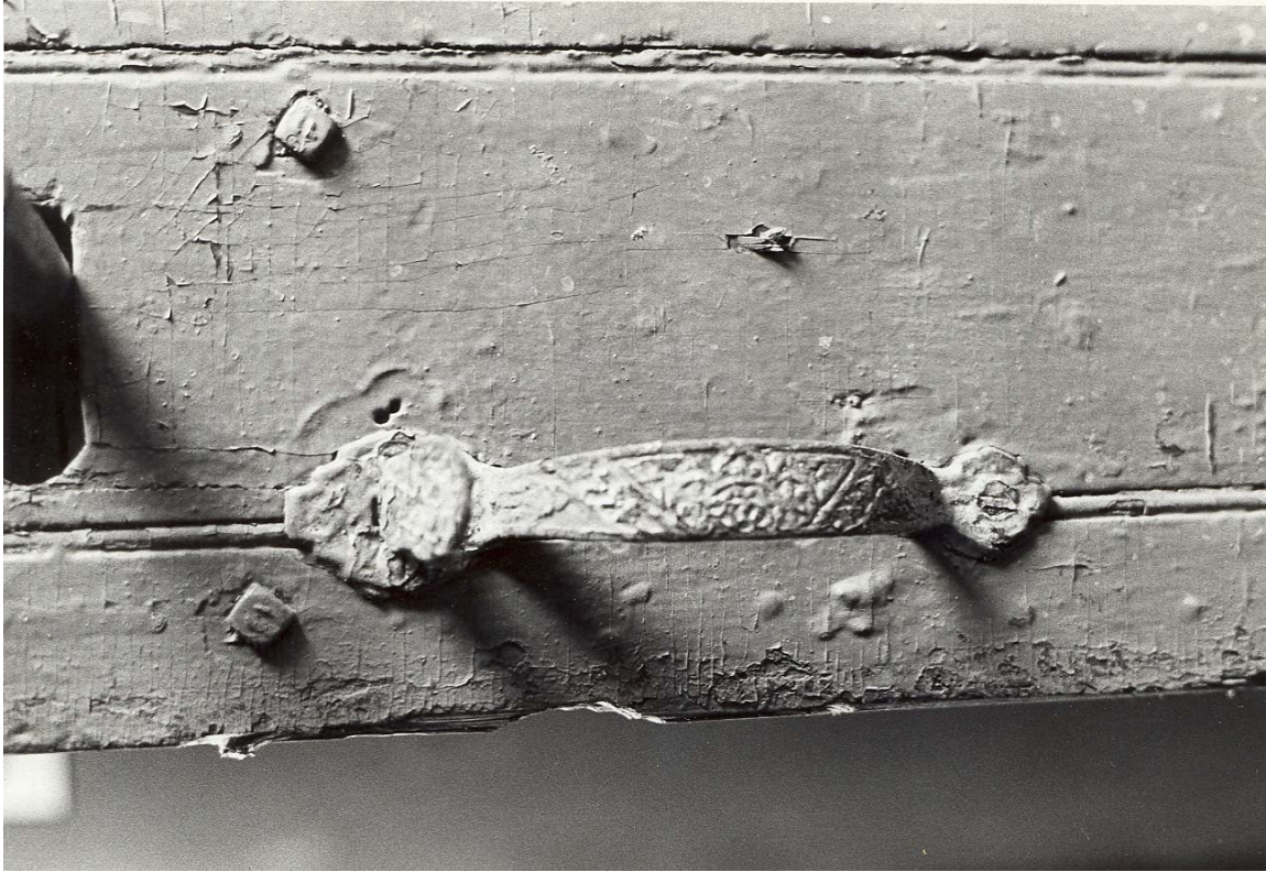
Figure 254. Dwelling interior: thumb latch on bulkhead side of cellar door to west bulkhead (1983).
