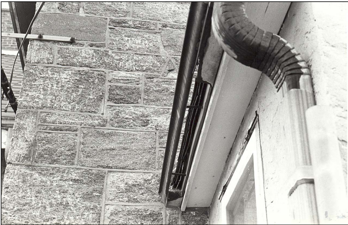
Figure 241. Dwelling exterior: east side of vestibule, gutter, and downspout (1982).
