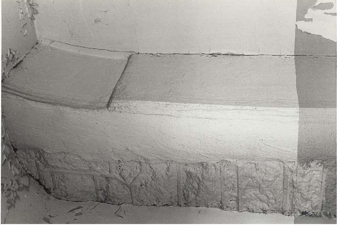
Figure 216. Dwelling interior: evidence for former covered passageway.
