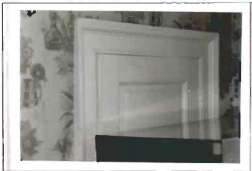
Photograph 5. D.R. Miller House - portion of an 18th century interior closet door and architrave, first floor, southeast room. Photo by Paula Reed. 6/91
