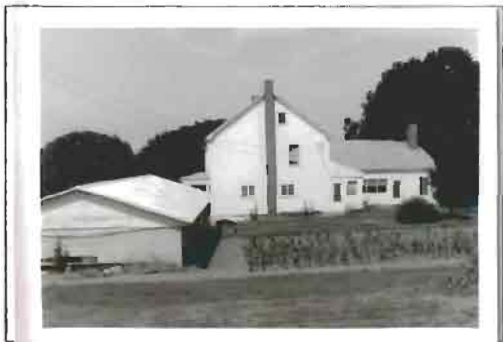
Photograph 3. D.R. Miller House, east elevation, west view. Photo by Paula Reed. 6/91
