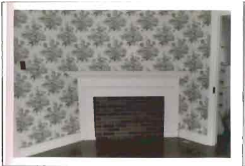
Photograph 7. D.R. Miller House. Former fireplace, northwest room, first story. Photo by Paula Reed. 6/91
