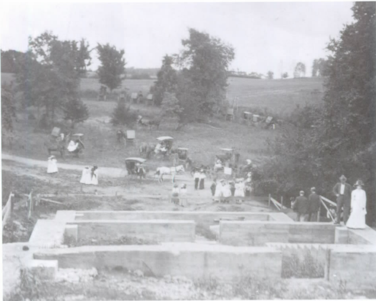
FIGURE 6. Construction of the Memorial Building Stairway, c. 1910.
