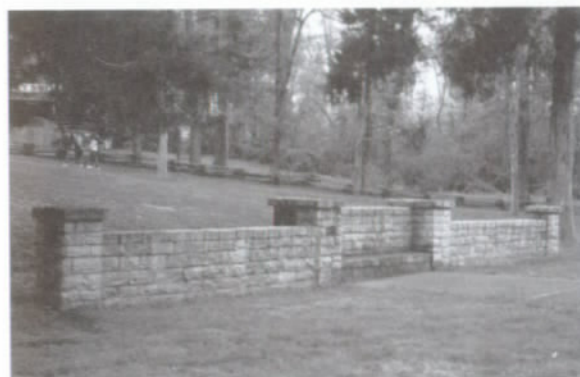
FIGURE 51. Lack of screening for the Nancy Lincoln Inn, 2001.
