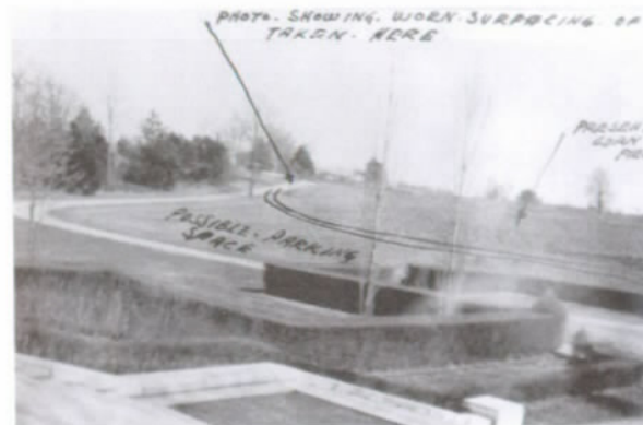
FIGURE 17. The entrance road and park landscape beyond, 1928.
