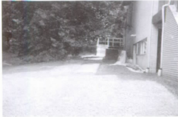
FIGURE 71. Asphalt walk at the rear of the Visitor Center, 2003.
