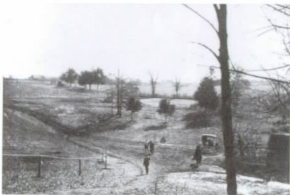
FIGURE 7. Construction shot showing agricultural setting of the site, c. 1910.
