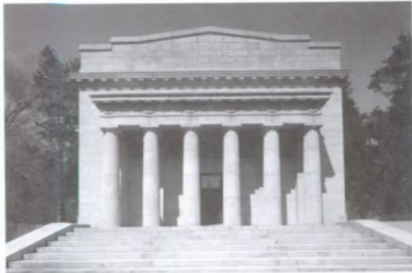
FIGURE 53. The Memorial Building, 1984.
