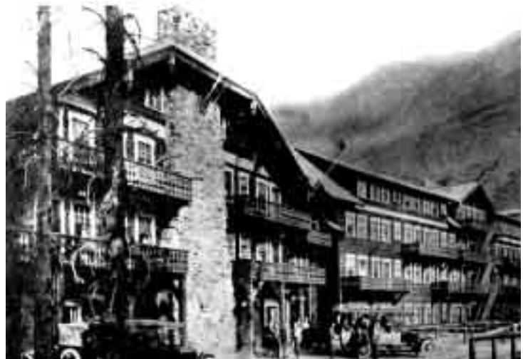
East side of hotel with tourists waiting to board the "Old White" touring buses. 1920 Note stone chimney at entry, flag pole supports, and balconies without extensive "add-on" supports (steel angles, cables, wood posts). Courtesy Glacier National Park Archives
