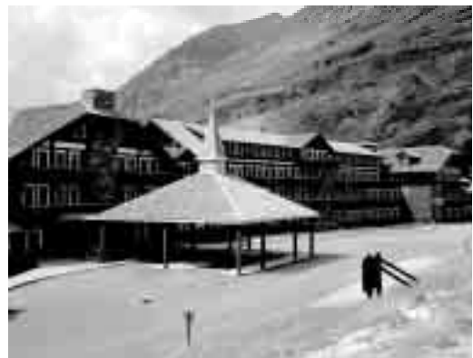
Porte Cochere added in 1957 to protect arriving and departing guests from the weather. Courtesy of Glacier National Park Archives
