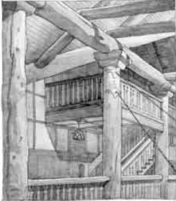
Painting of interior log structure: log columns with capitals, log beams and trusses. Original crafted balustrades. Patterned batten boards over Sackett board above wood wainscoting. Artwork Henry Sorensen 1999
