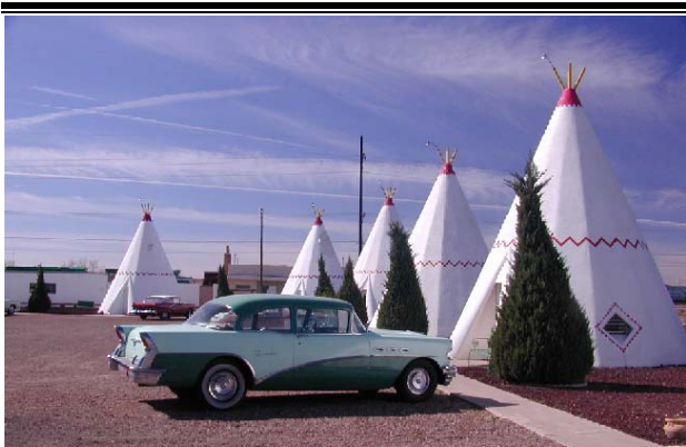
Wigwam Village No. 6, Holbrook, Arizona (1950). An example of a dramatic deviation from the normal tourist court tops, at least in the configuration of the individual units and drawing upon a western-related marketing theme in the postwar period along Route 66. Photo: Michael Cassity, 2004.
