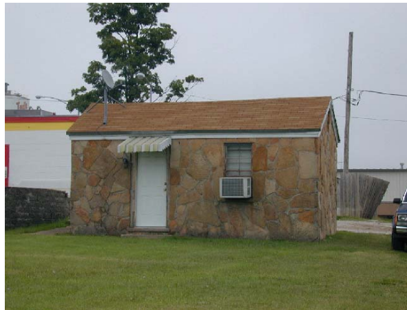
Sole remaining lodging unit of Wishing Well Motel in Springfield, Missouri, that served
