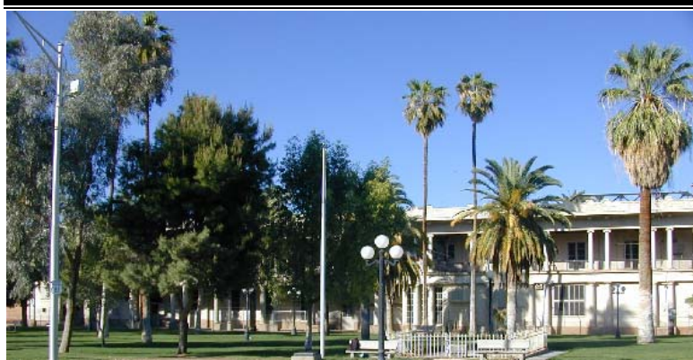
El Garces Hotel, Needles, California, one of the Fred Harvey chain of railroad hotels. Photo: Michael Cassity, 2002.
