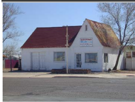
Conoco station (date unknown), Winslow, Arizona. Conforming to Conoco building requirements, this building is characterized by steeply pitched roofs, high, louvered vertical vent, and corbeled eave corners. The building has been modified, with the service garage apparently added later, but is especially notable for retaining its wooden doors in the service bay. Photo: Michael Cassity, 2004.
