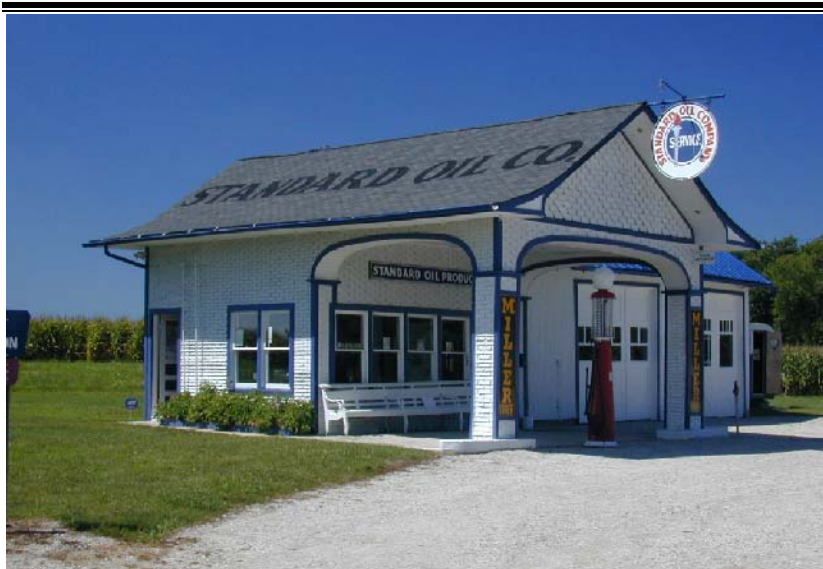
Odell Standard Station, Odell, Illinois (1932). This station, built to Standard Oil Company requirements, has been restored to its original appearance, including, however, the service bays added in 1940. Although the drive has been altered, the original configuration enabled the pumps to be accessed on both sides, with one lane under the canopy and the second outside. A café once was located next to the service station. An example of a house with canopy station, with additional service bays, the evolution of this gasoline station reflects both changing corporate identities (in 1940 it was selling Phillips 66 products and later on it sold Sinclair) and service station functionality. Photo: Michael Cassity, 2004.
