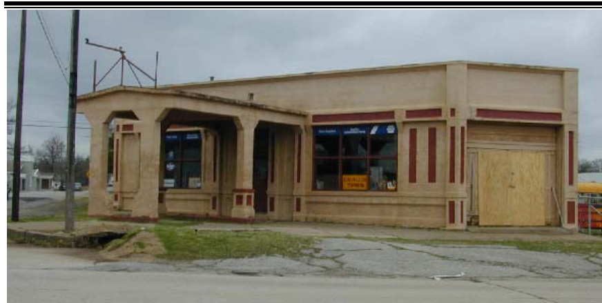
Hicks' Garage and Service Station, Depew, Oklahoma (c. 1922). An elaborate service station that predated U.S. 66, this is an example of the property type Gasoline / Service Stations. A house with canopy station in general form, it represented several distinctive features with the unusual configuration of the office/store and service area, but it is especially notable because of its individualized construction that does not conform to a larger chain or corporate branding effort. The lanes at the pump islands would not long be able to handle the cars and trucks because of their narrow dimensions. Photo: Michael Cassity, 2002.
