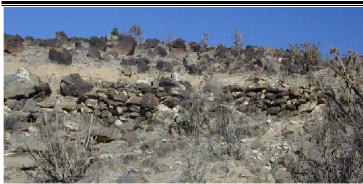
Retaining wall on La Bajada allowing motorists on U.S. 66 to gain a slightly better hold on the road. Photo: Michael Cassity, 2004.
