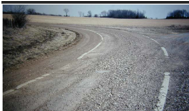
Road turn of U.S. 66 near Miami, Oklahoma where the corner is a 90 degree turn to follow the section lines. This is a section of the highway where the roadbed was only nine feet wide, with concrete curbs on each side. Photo: Michael Cassity, 2002.
