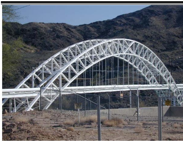
Bridge over the Colorado River at Topock, Arizona (1916), a three hinged steel arch bridge, that served the National Old Trails Road before it became an important Highway 66 bridge. No longer carrying vehicular traffic, its use is restricted to supporting a pipeline. Photo: Michael Cassity, 2004.
