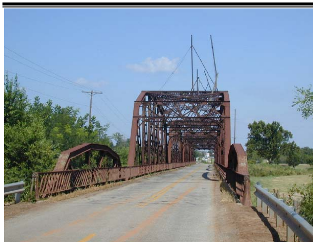
Lake Overholser Bridge, Oklahoma City (1924-1925) replaced a ferry across the North Canadian River. The bridge is a combination of camelback Warren pony trusses on each end and four Parker through-trusses between. Photo: Michael Cassity, 2003.
