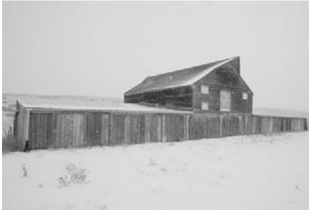
During the fall of 2003, the Service, in partnership with DOE, stabilized the barn and rebuilt the two wings.
