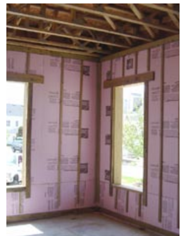
FIGURE11: Masonry Walls with Interior Rigid Insulation
