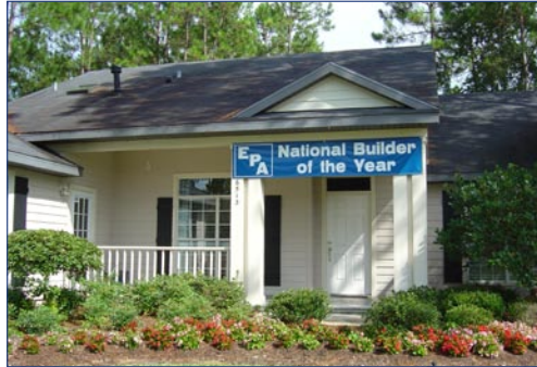
Atlantic Design, a Building America partner, was recognized as a 2000 EPA Builder of the Year for its quality energy-efficient construction.
