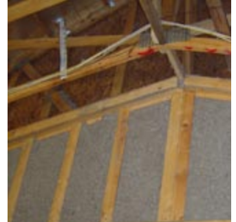
Blown-in wall insulation
