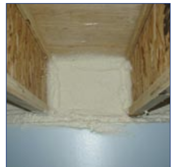
Spray-in foam insulation. Soy-based foams are now available (Photo: Building Science Corporation)
