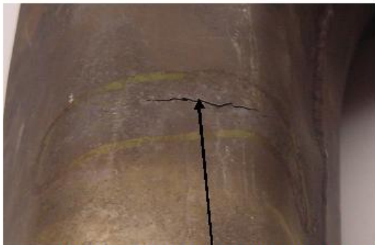
Crack through forward side of tailpipe.
