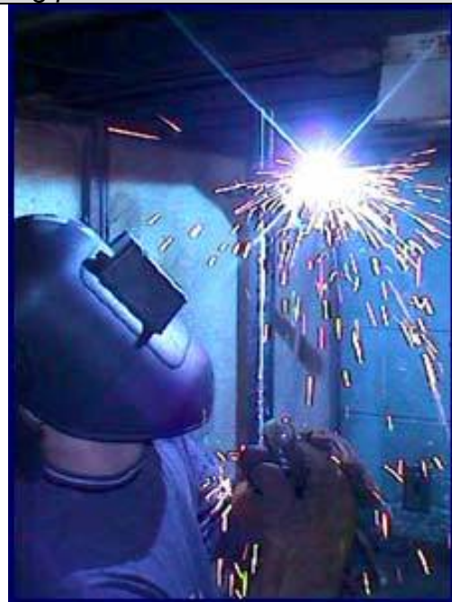
Figure 6 Welding above shoulder height
