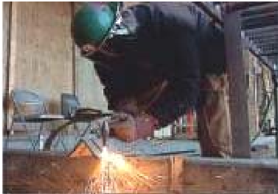
Figure 34 Before: Welder is bent over work piece
