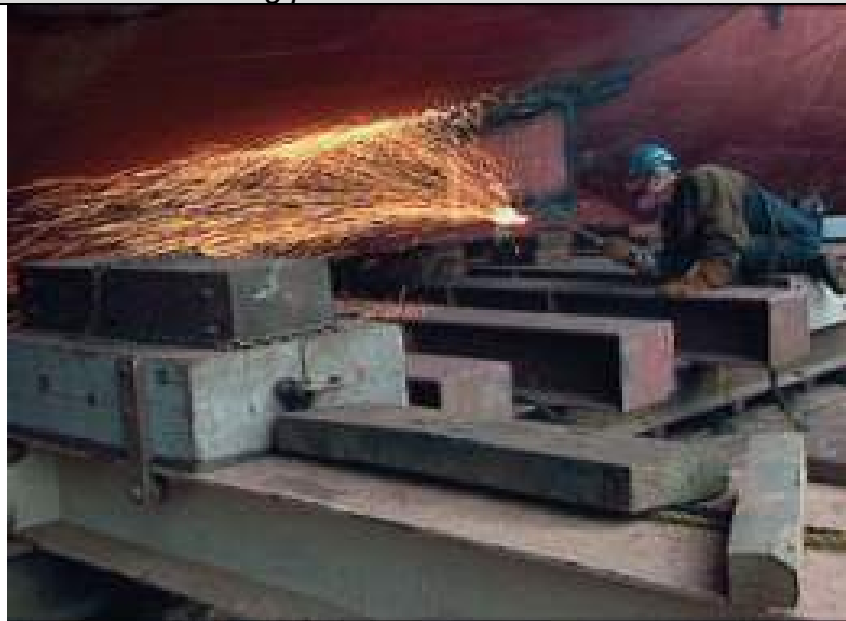
Figure 7: Welding in constrained spaces
