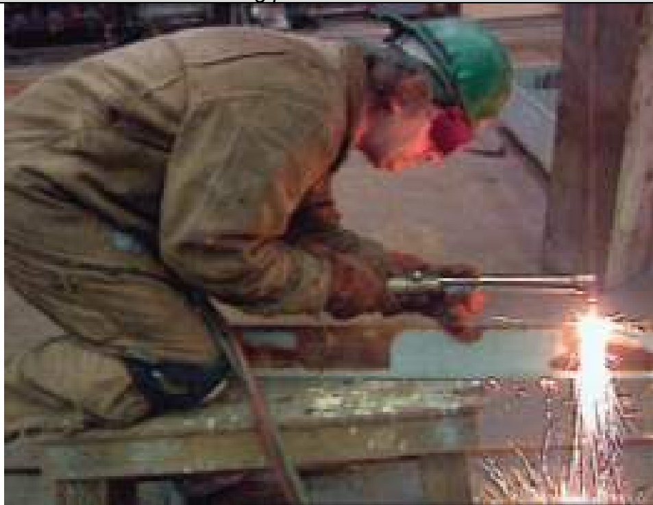
Figure 9: Working with the back bent forward
