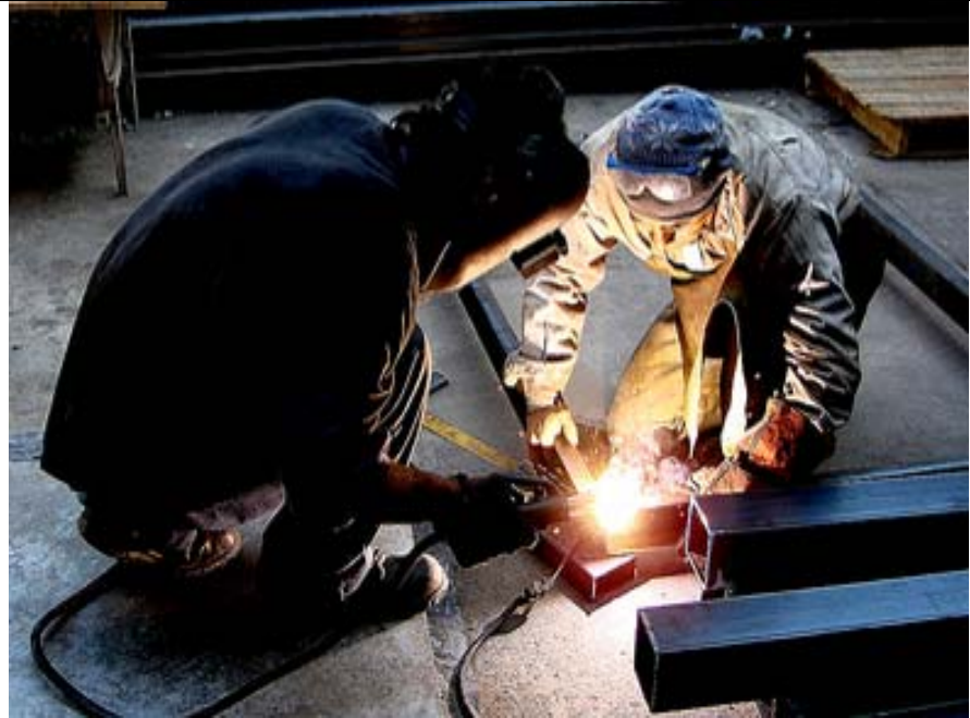
Figure 5: Welding at ground level
