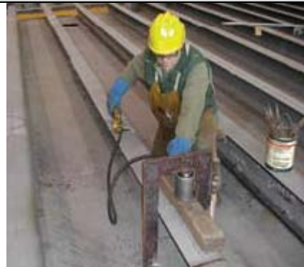
Figure 48: Welder using manual clamp method
