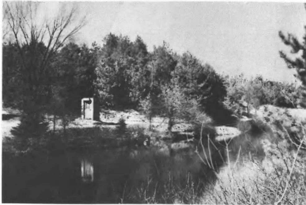
Records of streamflow are obtained from gaging stations such as this on the Huron River at Milford. FIG. 33
