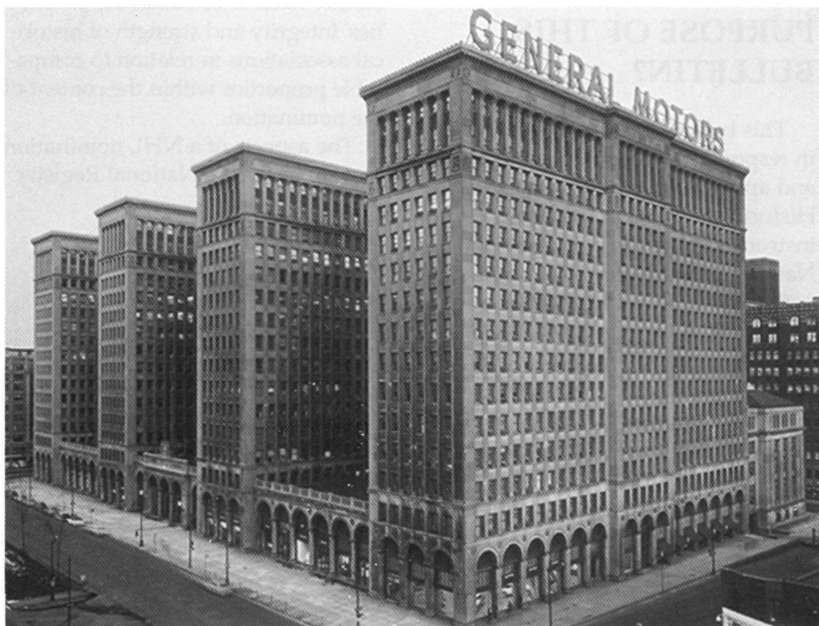
Albert Kahn designed this fifteen-story structure with its clearly defined base, shaft and attic story. Completed in 1923, the tripartite vertical arrangement was typical of tall building design at that time.
