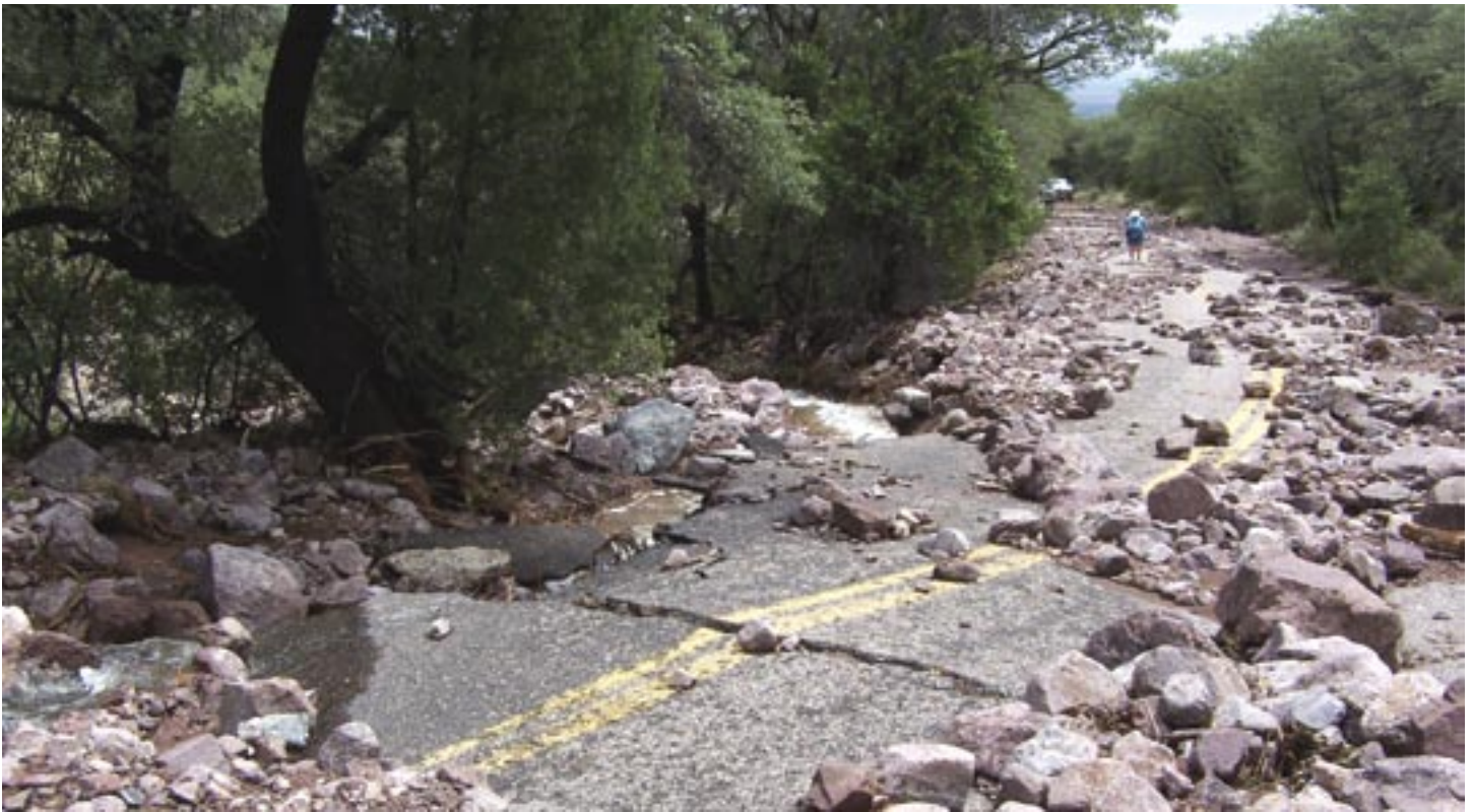
Heavy summer rains caused flooding at Coronado National Memorial where parts of a paved road were washed away and the unpaved road to Montezuma Pass was made impassable by boulders and other debris. NPS PHOTO BY CARLOS HERRERA
